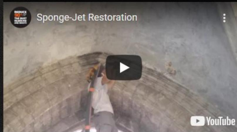
Sponge Media™ cleaning and restoration products provide professionals with surgical-like control for a wide range of cleaning and restoration work. The media's engineered capabilities range from gentle cleaning to micro-abrasion, with Sponge-Jet Feed Unit™'s propelling the media at pressures so low, one can clean paper.
