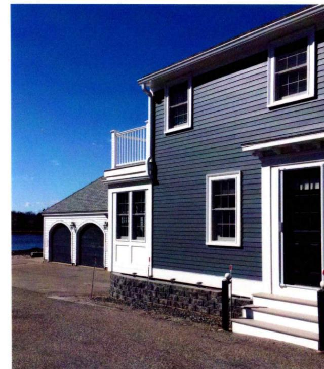
HARD-PLANK LAP SIDING AT EXIST. BUILDING
