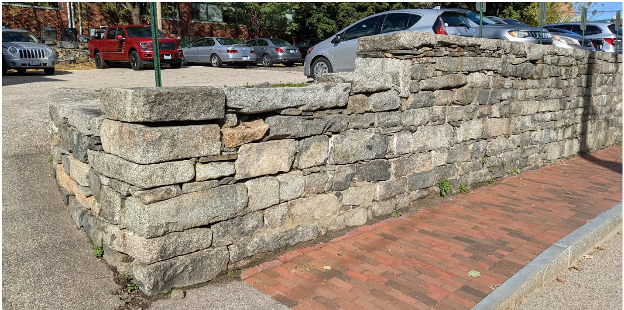
STONE WALL - EXISTING CONDITIONS
