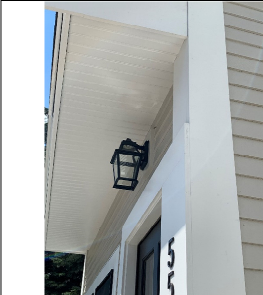
Door trim overlaid on corner board
