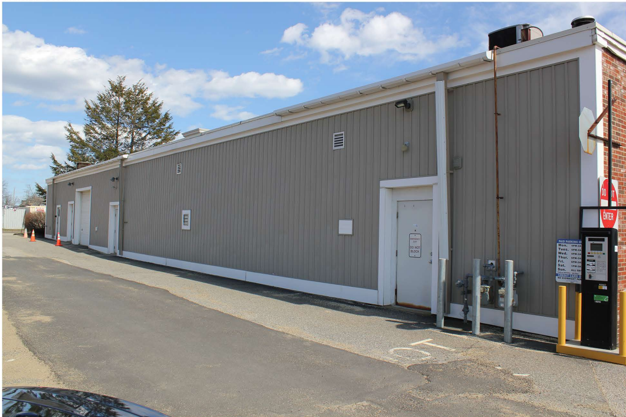
ELEVATION FACING RAILROAD TRACKS
