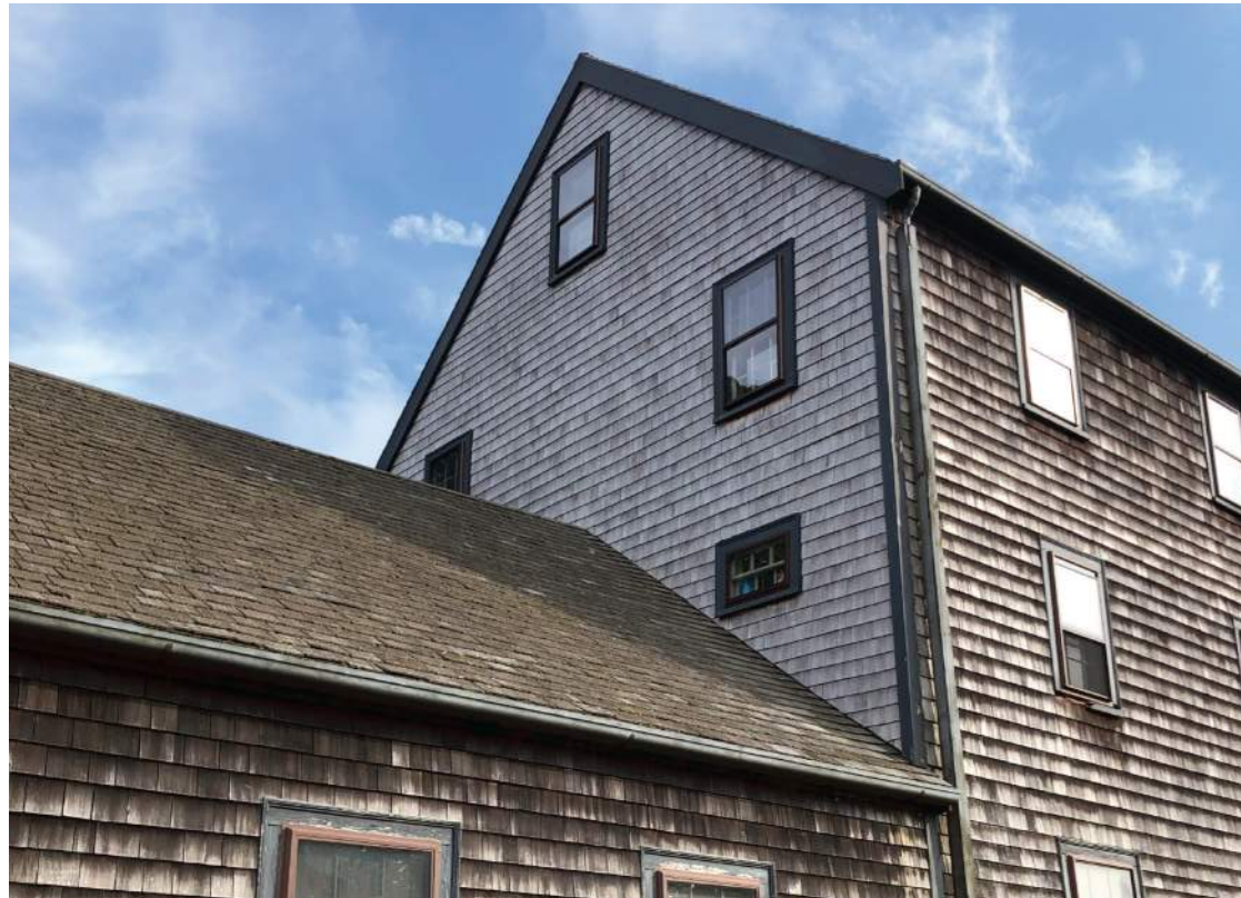
Shaw to Lean-to interface (exterior)
