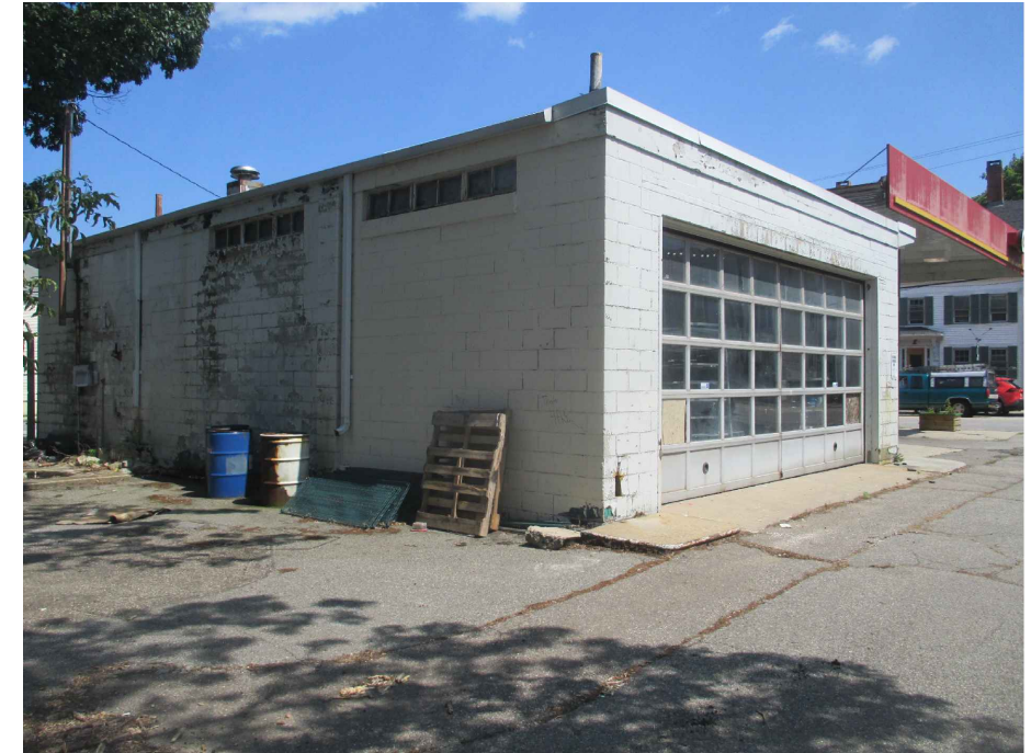
EXISTING NORTH WEST BUILDING CORNER
