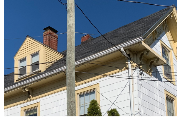
Original chimney, capped at ridge
