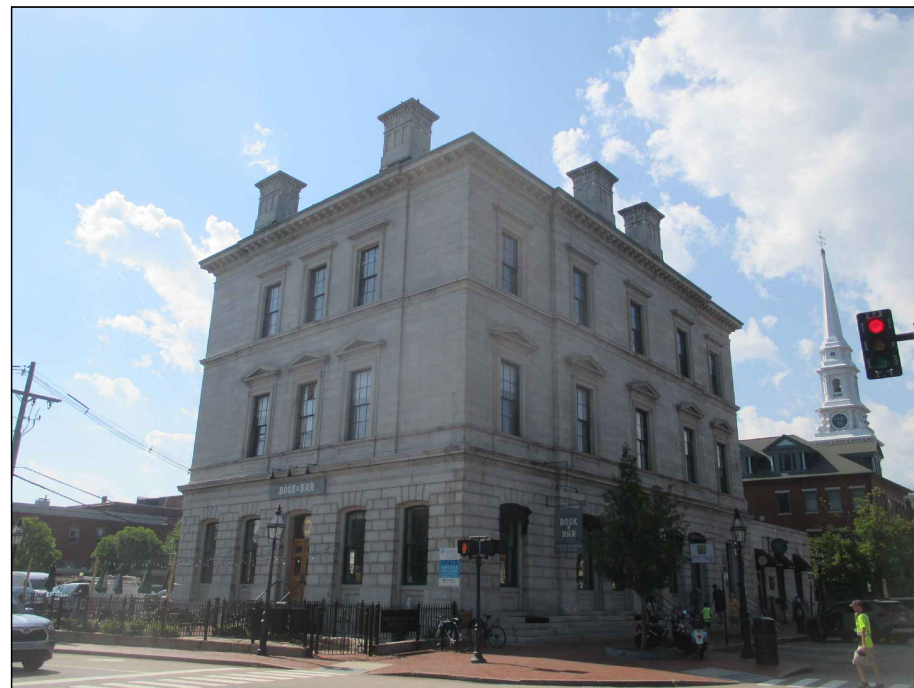
EXISTING SOUTH EAST BUILDING CORNER
