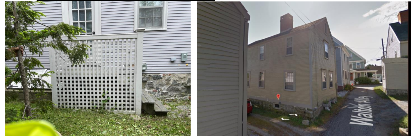
Rear Elevation and Streetscape View
