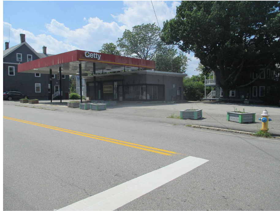
EXISTING VIEW FROM SOUTH EAST
