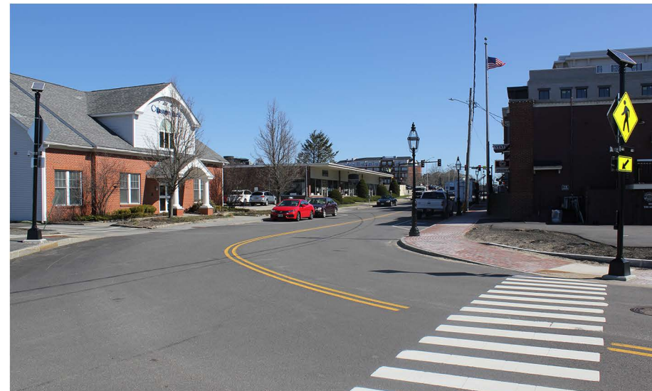
H. VIEW OF SITE FROM THE CORNER OF BRIDGE STREET
