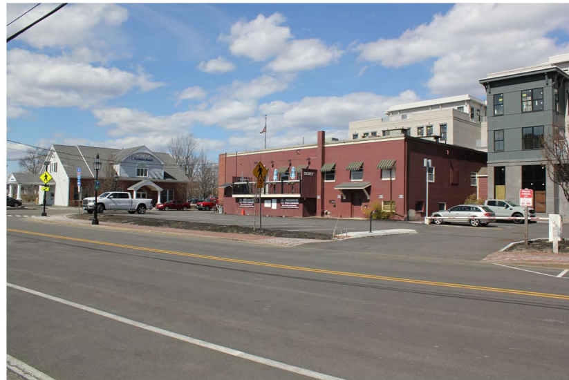
G. VIEW OF THE SITE FROM BRIDGE STREET
