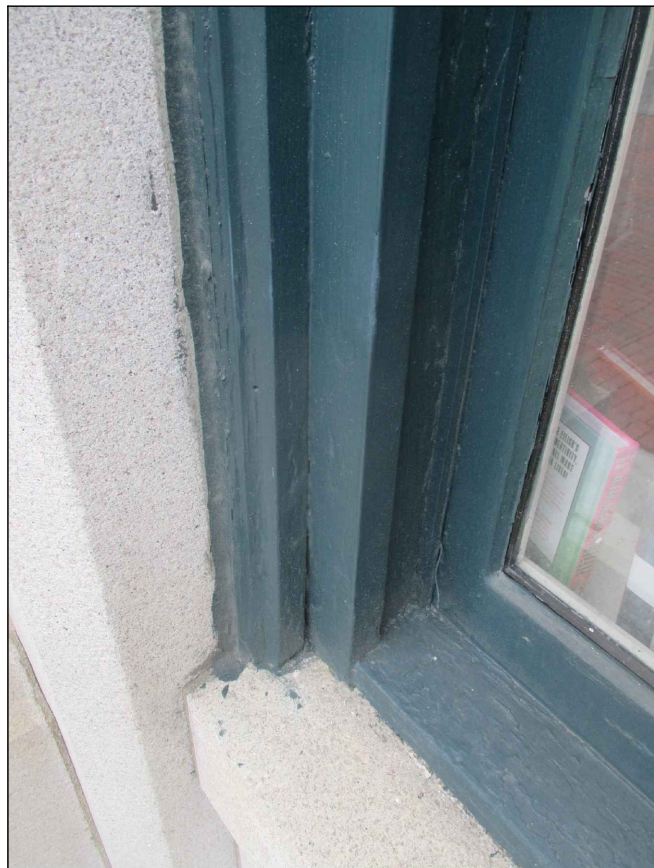
INSULATED GLASS WITH WOOD BRICK MOULD AND WOOD SILL
