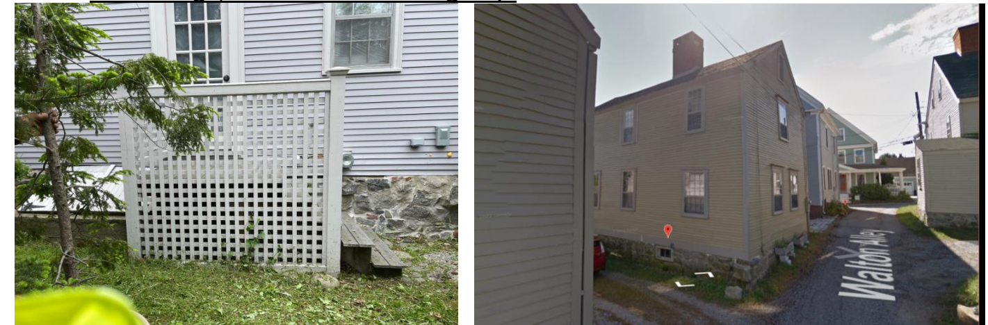
Rear Elevation and Streetscape View
