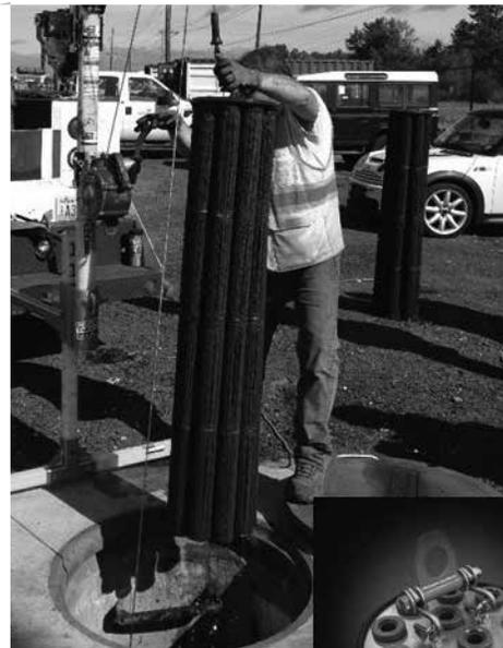
Cartridge Removal & Lifting Device
