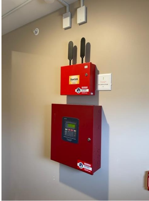
Figure 7. Fire Alarm Panel
