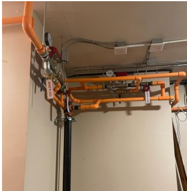
Figure 6. Orange CPVC Piping
