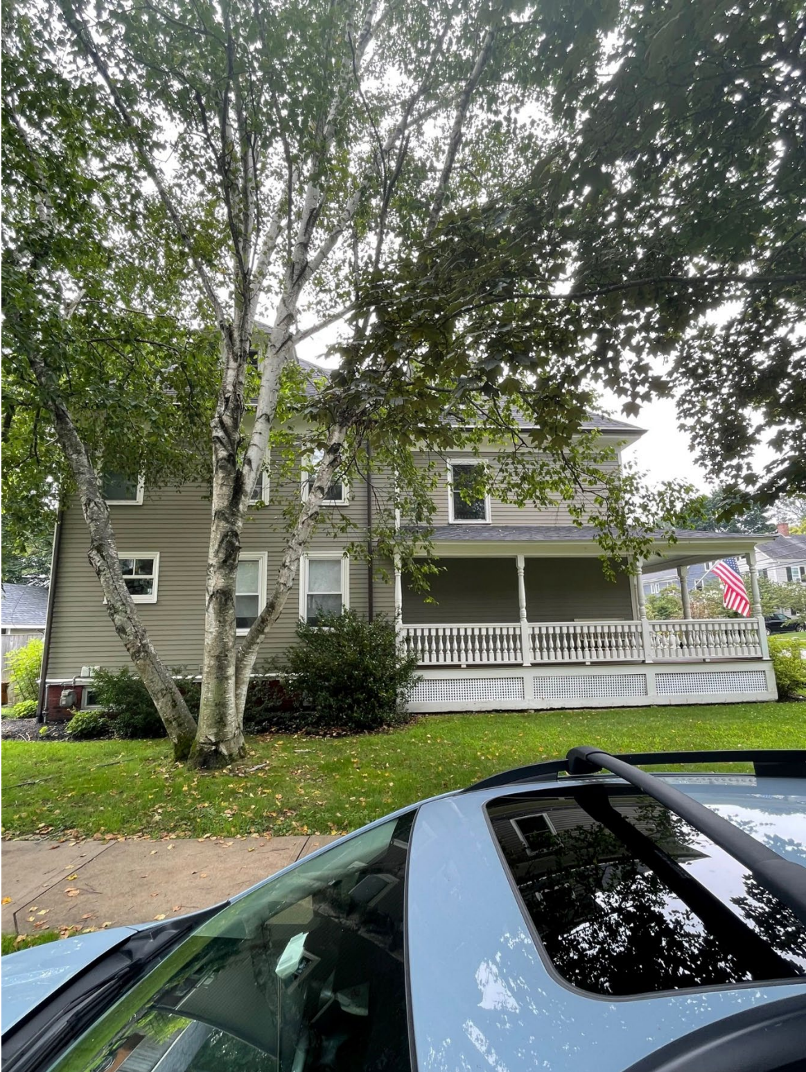
Left Side Yard View of Property (Lincoln Ave)
