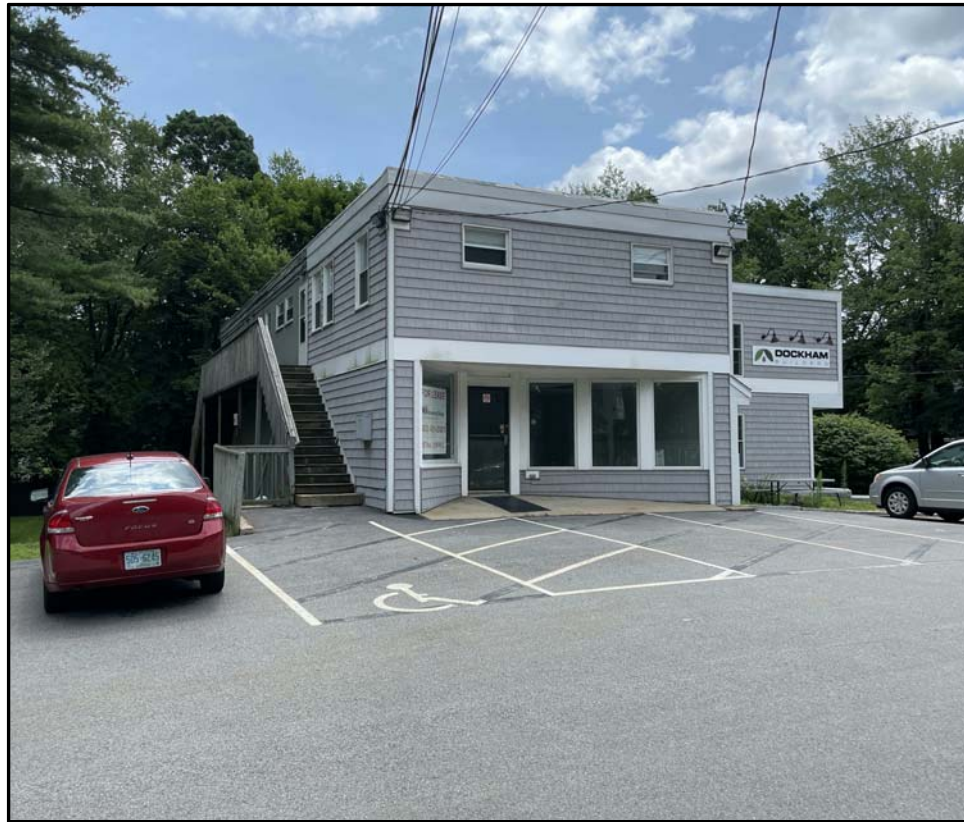
2059 LAFAYETTE ROAD LOOKING SOUTH
