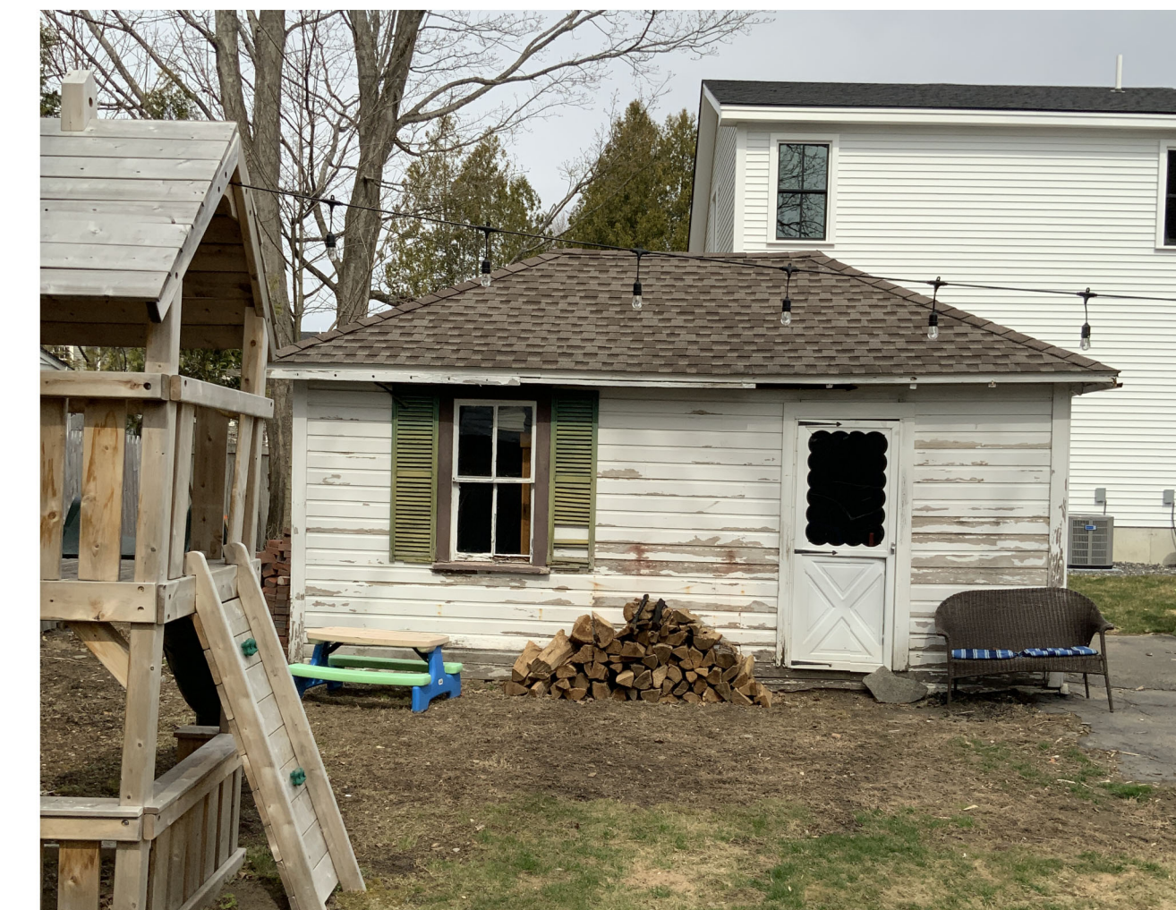
EXISTING BACK GARAGE PHOTO
