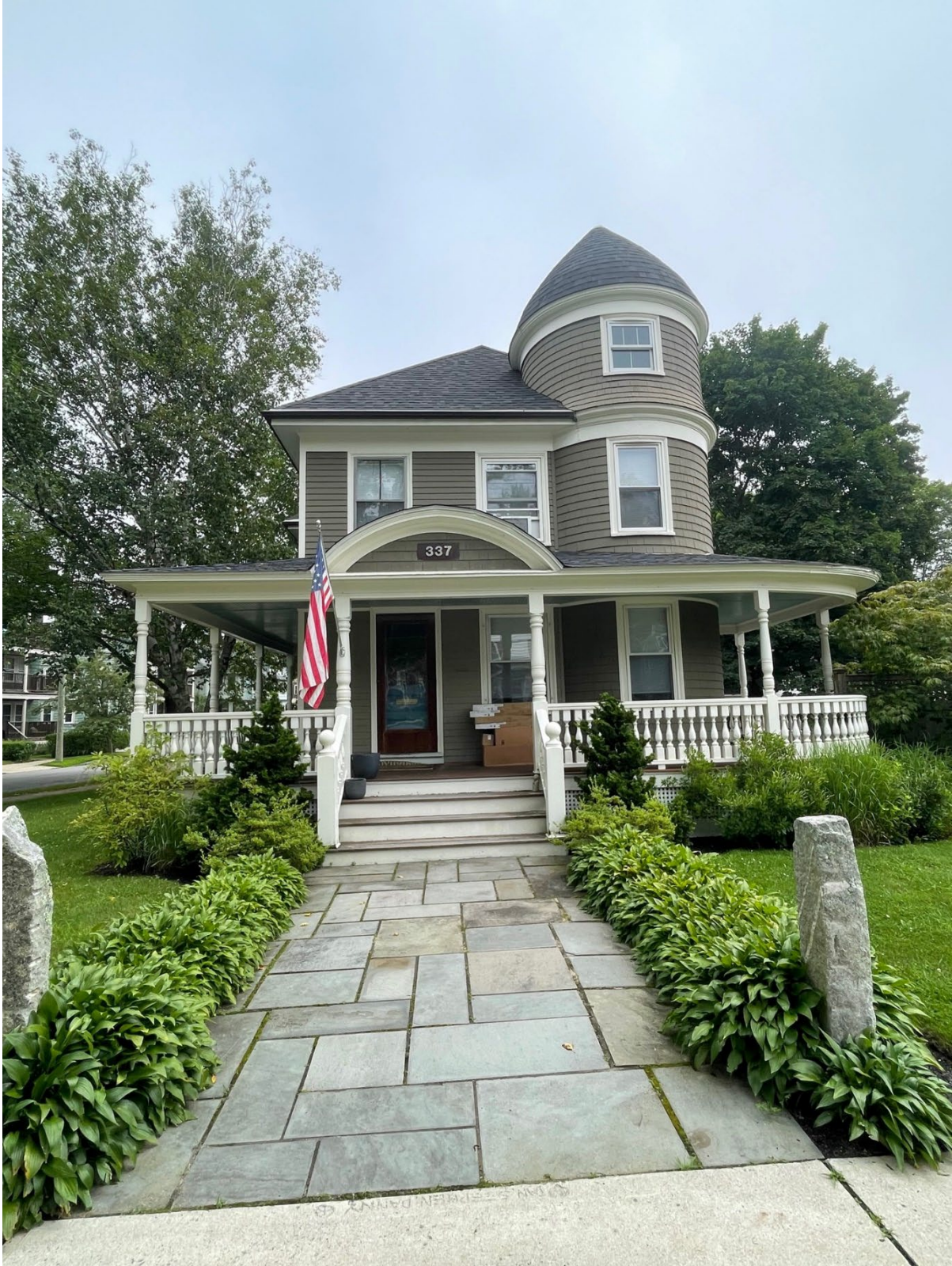
Front View of Property (Richards Ave)
