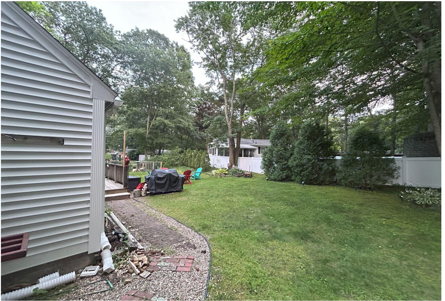
Property Photo #5 View adjacent to Breezeway Wall looking SouthEast
