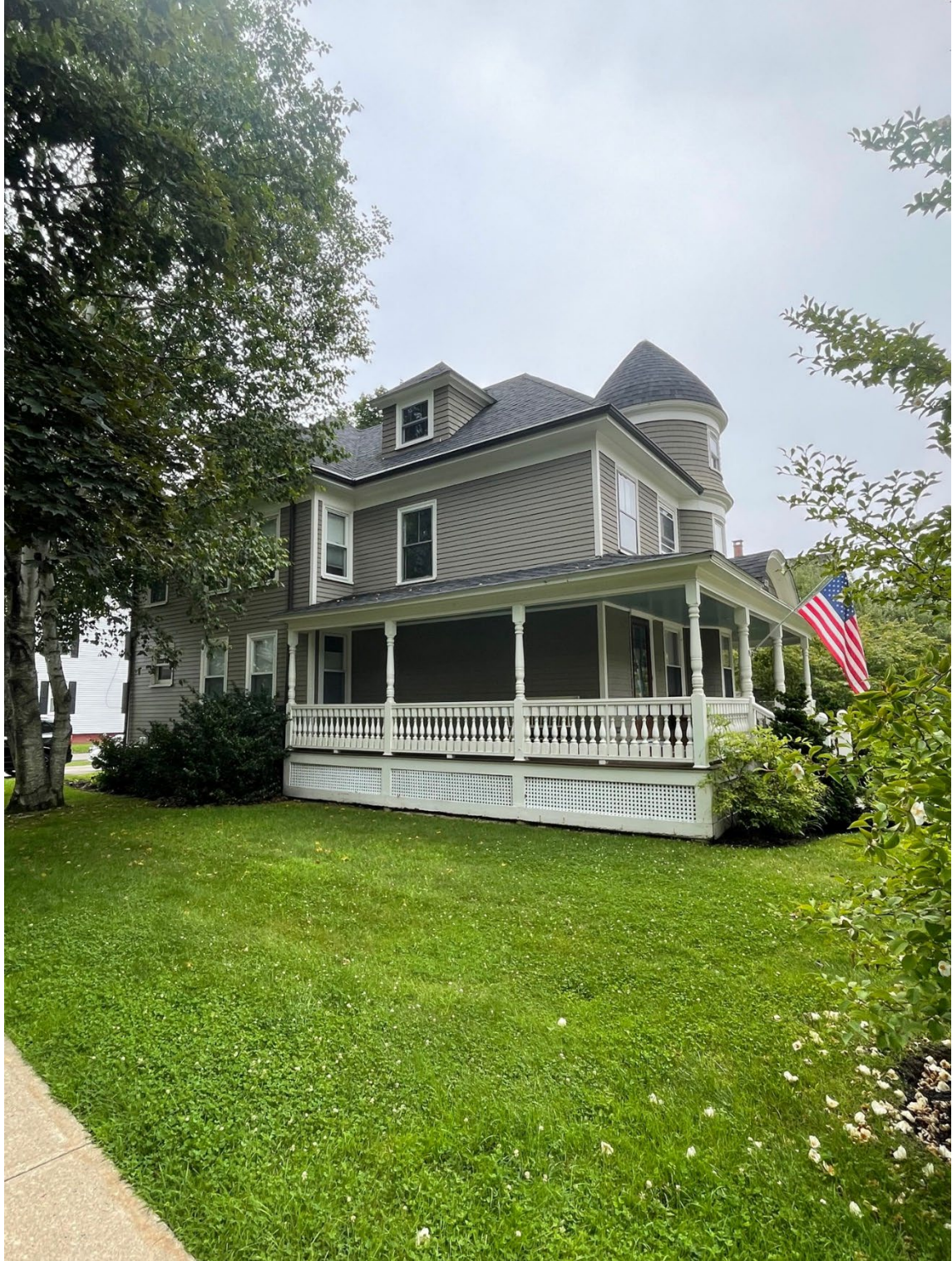
Front - Left View of Property (Intersection of Richards & Lincoln Ave)
