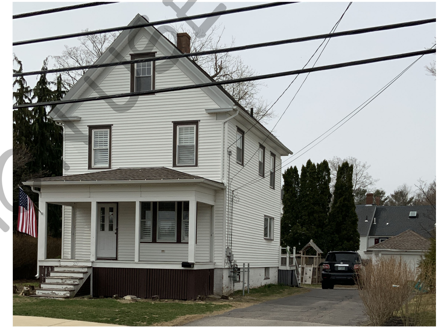
EXISTING RIGHT SIDE PHOTOS
