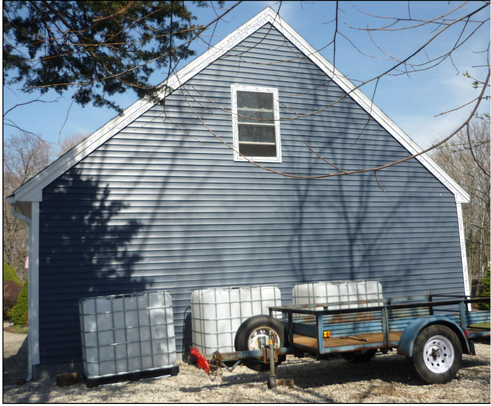
RIGHT SIDE GARAGE
