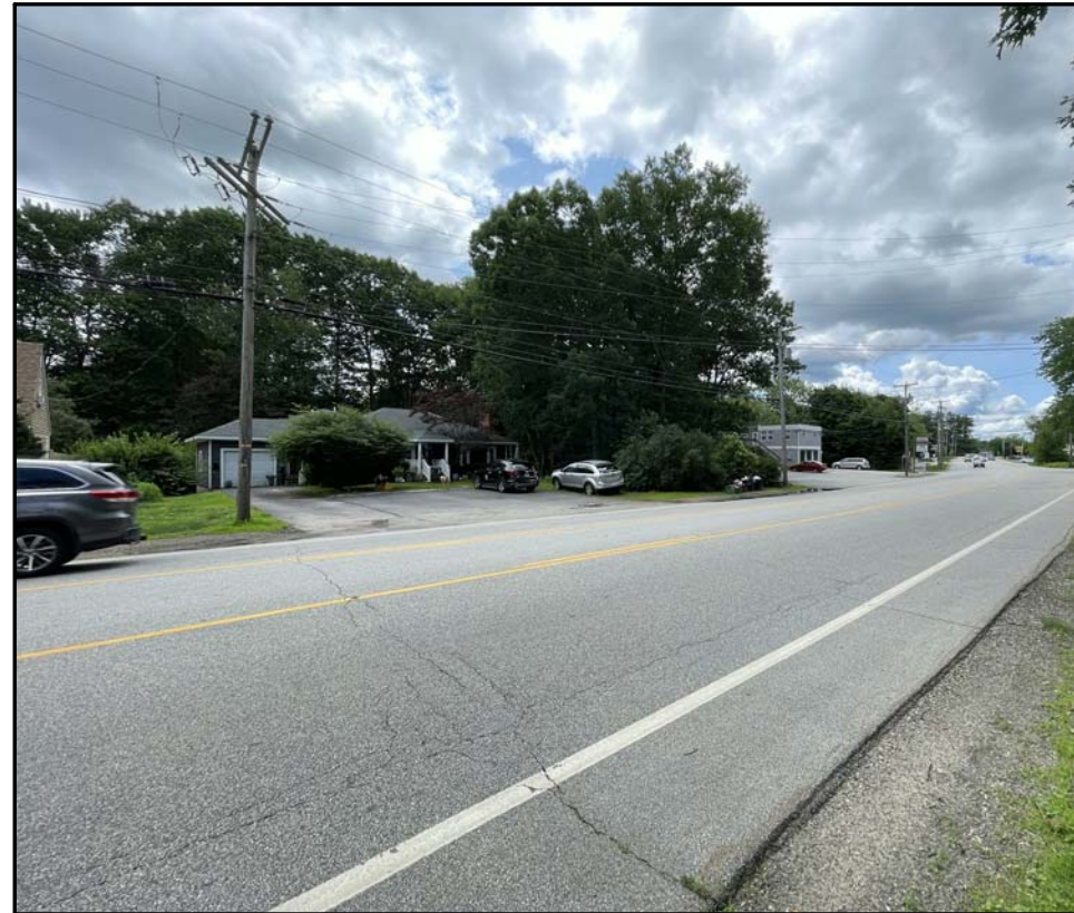
BUILDING APPROACH FROM NORTH
