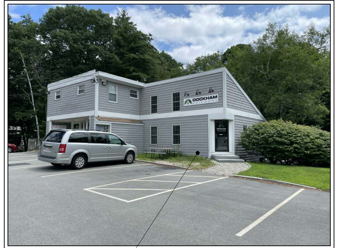
2059 LAFAYETTE ROAD PORTSMOUTH, NH 03801
