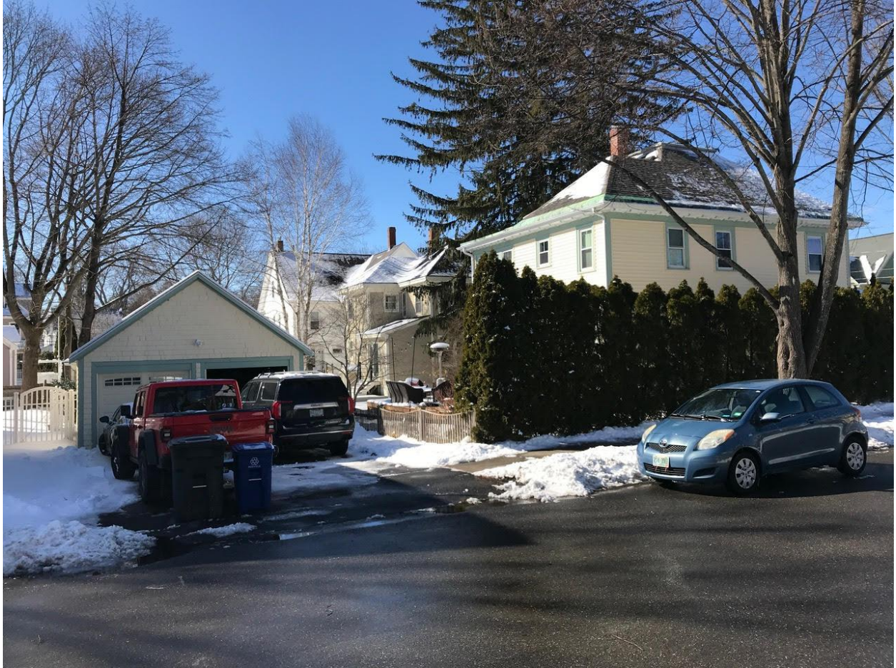
Non-Conforming Garage / Rear View of Property
