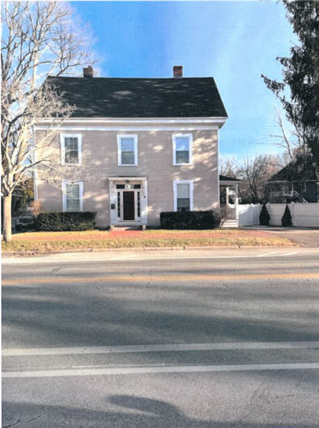
729-733 Middle Street Condominiums
