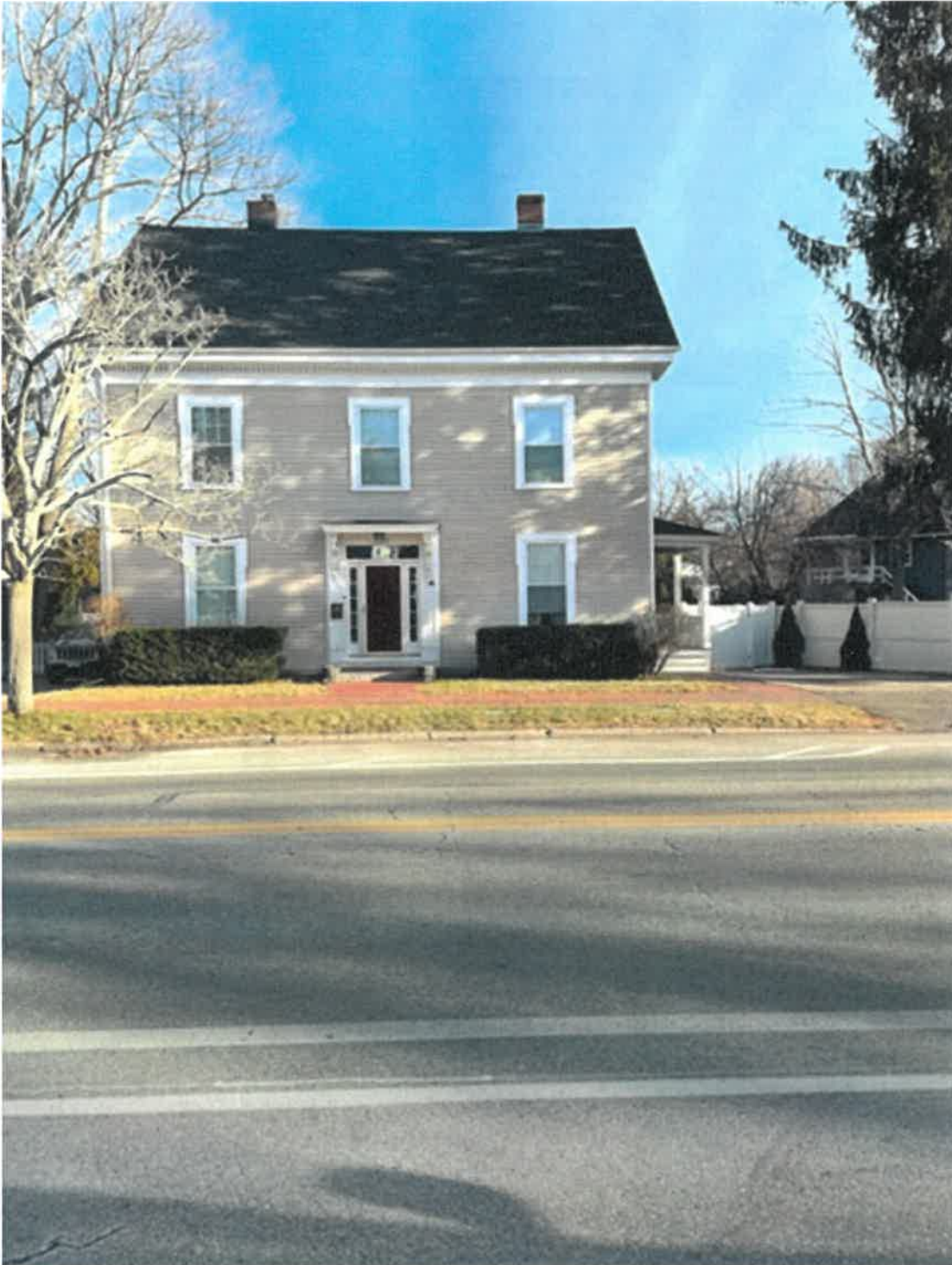
729-733 Middle Street Condominiums
