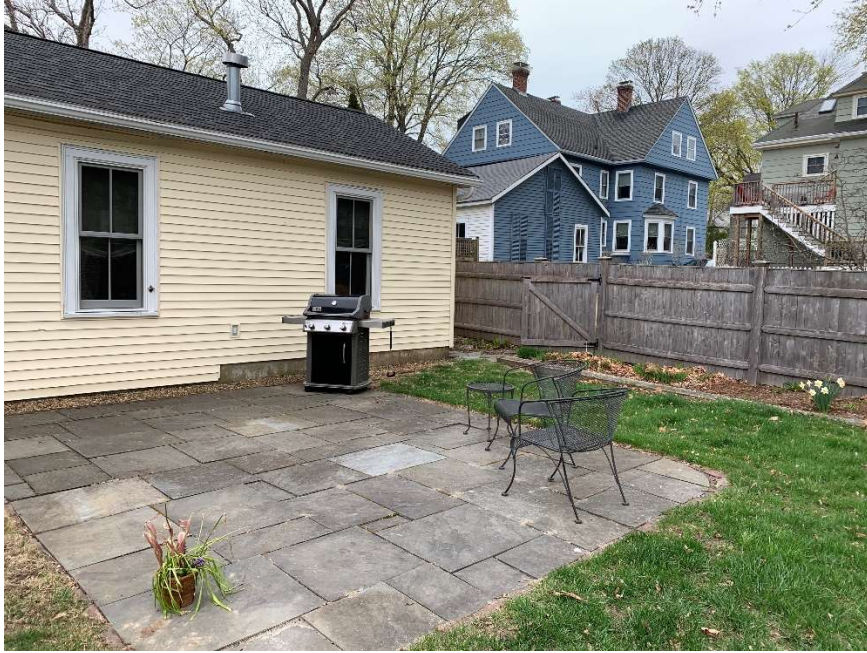
Side view of property indicating that alternate location for heat pump unit would be adjacent to patio and near fence gate.
