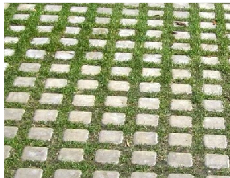
DRIVEWAY PAVERS GRANITE SQUARE POROUS 1/4" GRASS INSTALL
