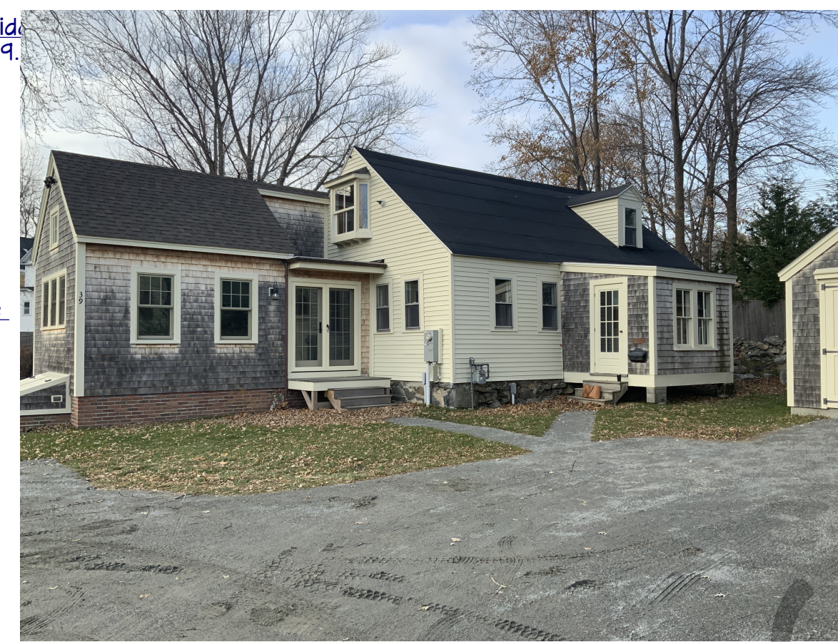
EXISTING FRONT HOUSE
