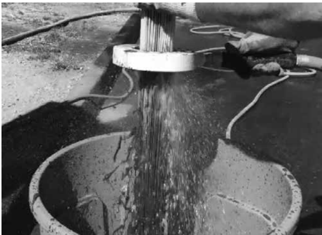
Vacuuming Sump Through MAW
