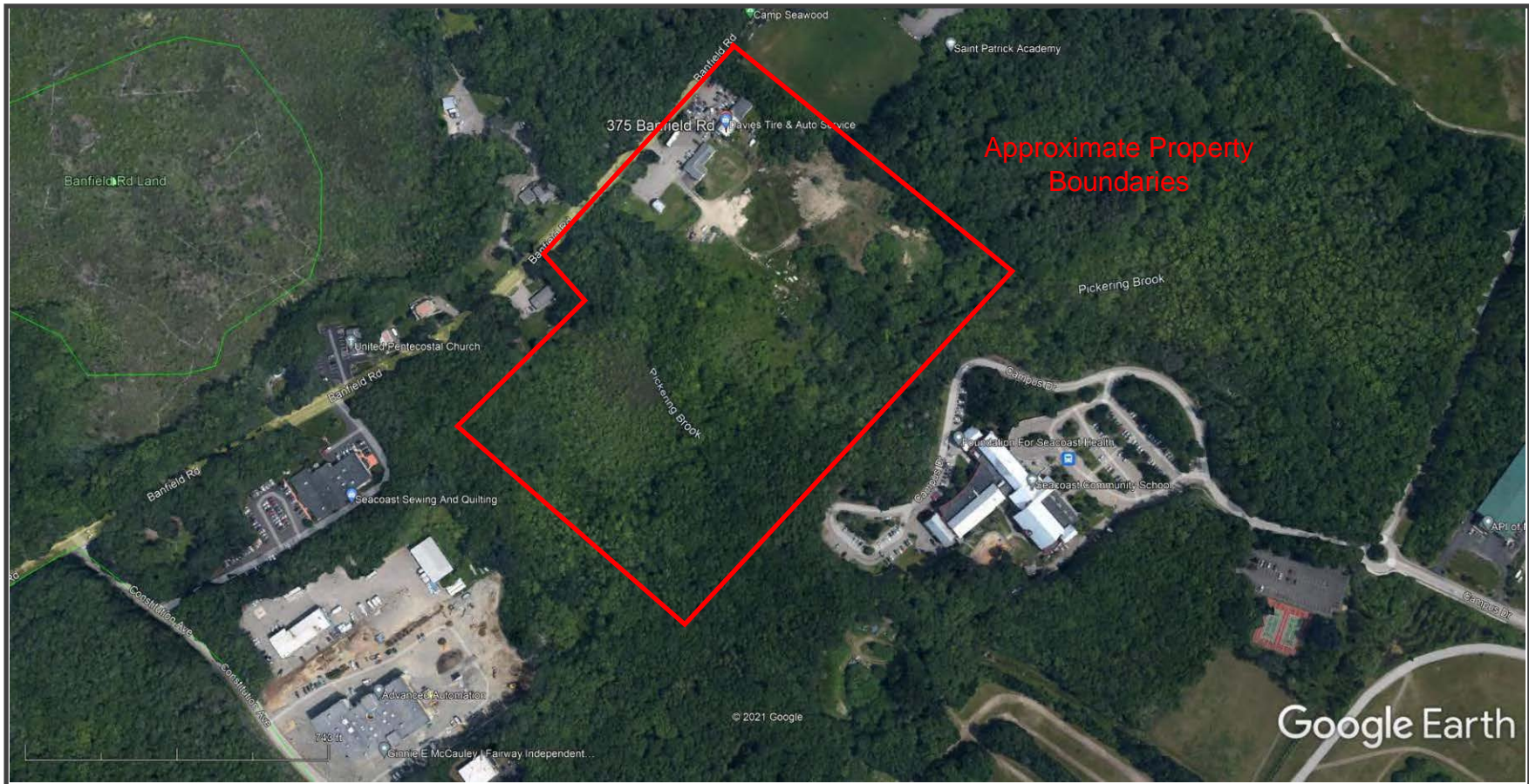
FIGURE 1 SITE AERIAL VIEW 375 Banfield Road, Portsmouth, New Hampshire
