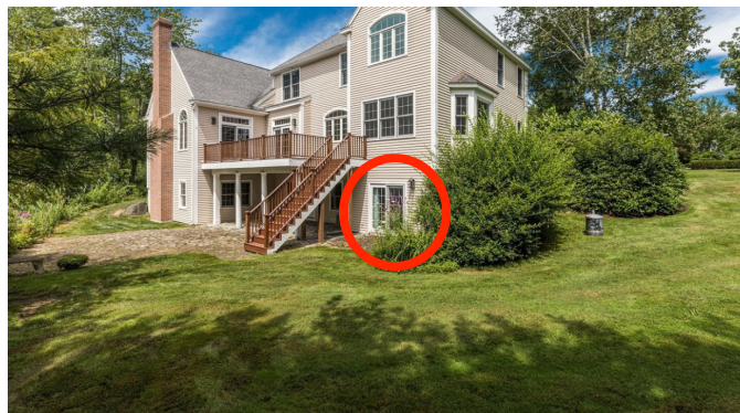
Exhibit #5, Walkout Basement Doorway
