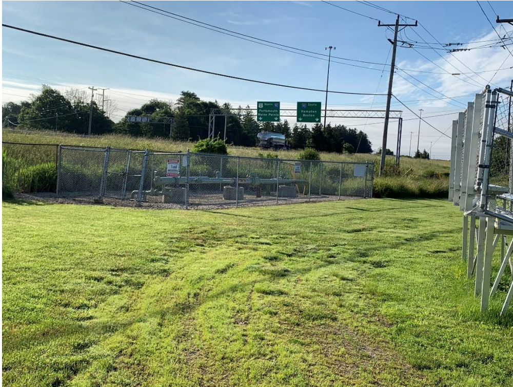
Photo 1: View looking Northeast towards the station on “manmade wetlands”
