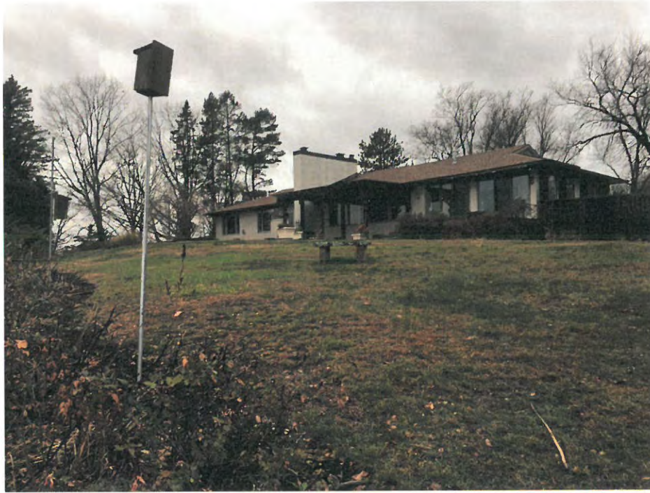
Photo #11: Looking northwesterly at existing residence to be replaced. November 23, 2020
