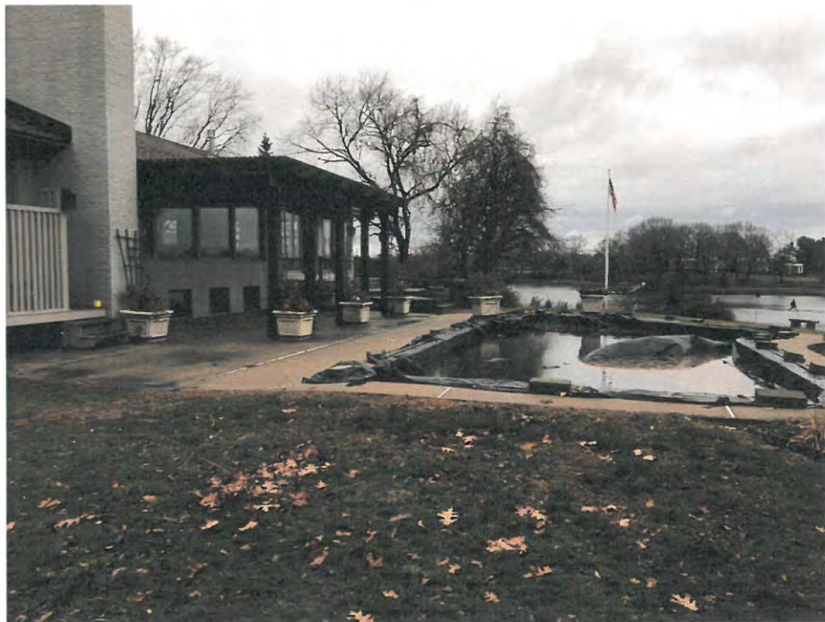
Photo #8: Looking northeasterly at pool and residence to be replaced. November 23, 2020
