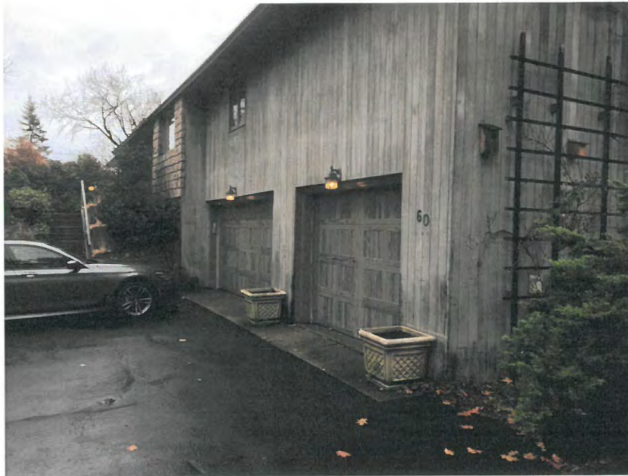
Photo #4: Looking easterly at existing residence to be replaced. November 23, 2020
