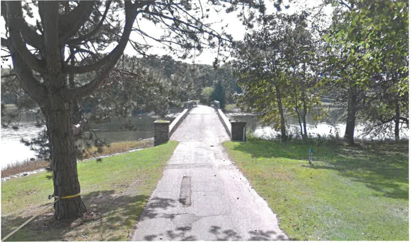
Photo 5. A final view of the bridge approach on Lady Isle to be replaced as well as a portion of upland.
