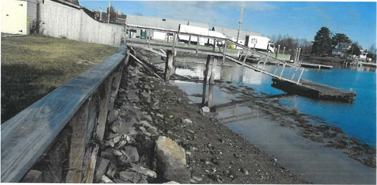
Photo 5 – Looking northerly along the retaining wall along the Piscataqua River - January 11, 2023.
