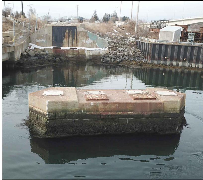
BRIDGE PIER 14 LOOKING SOUTHWEST (C3)
