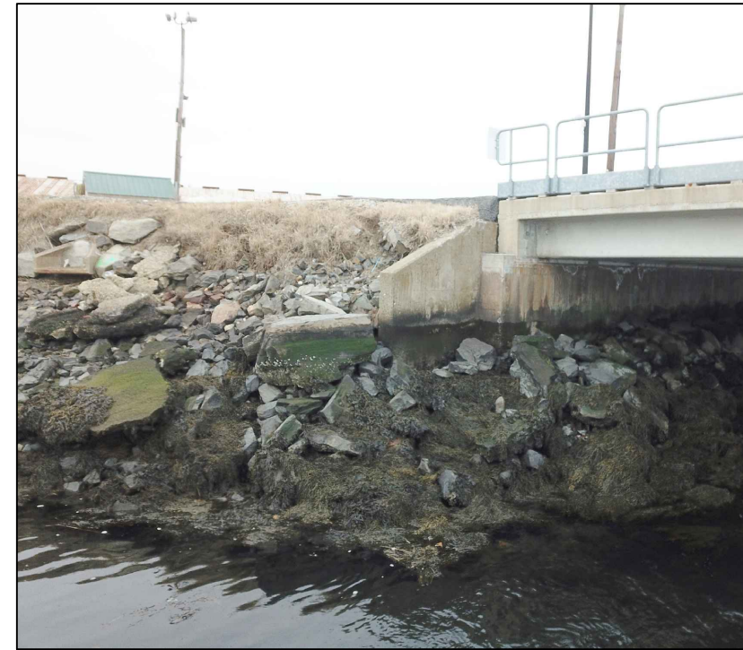
MAIN WHARF - BRIDGE ABUTMENT LOOKING WEST
