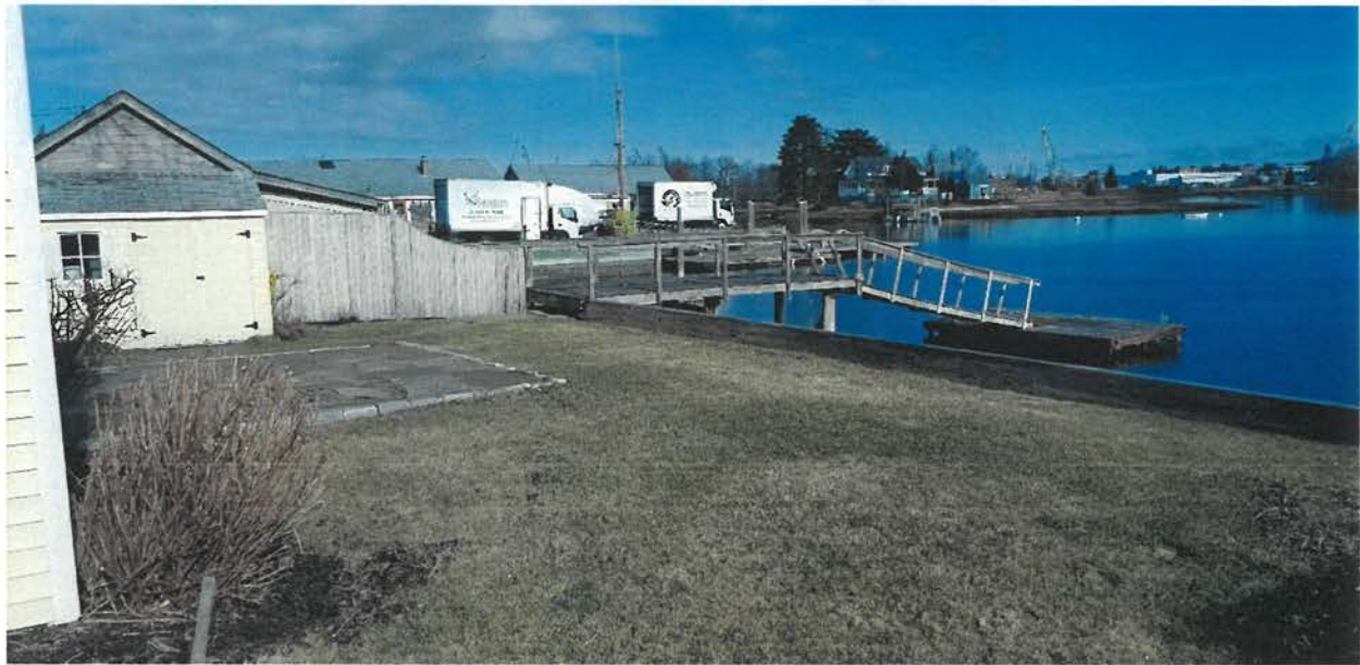
Photo 6 – Looking northerly at the water, backyard, dock, and stone patio - January 11, 2023
