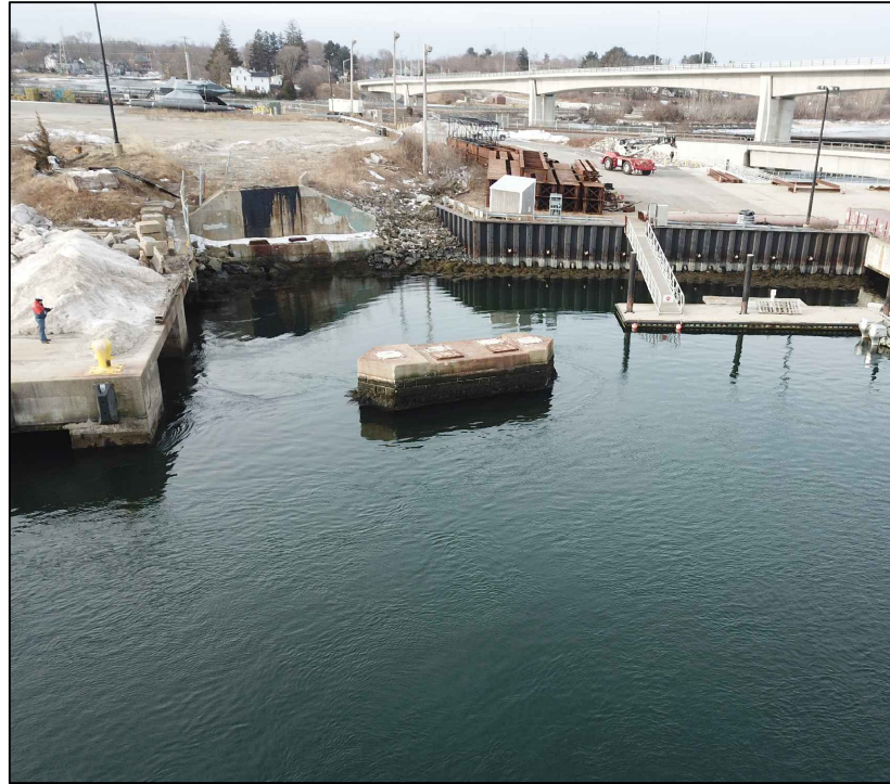
NORTH WHARF EXTENSION LOCATION LOOKING SOUTHWEST (C1)
