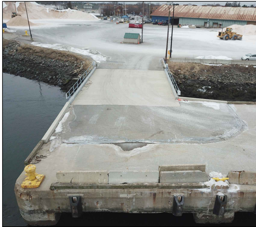
MAIN WHARF - SOUTH ACCESS BRIDGE LOOKING SOUTHWEST
