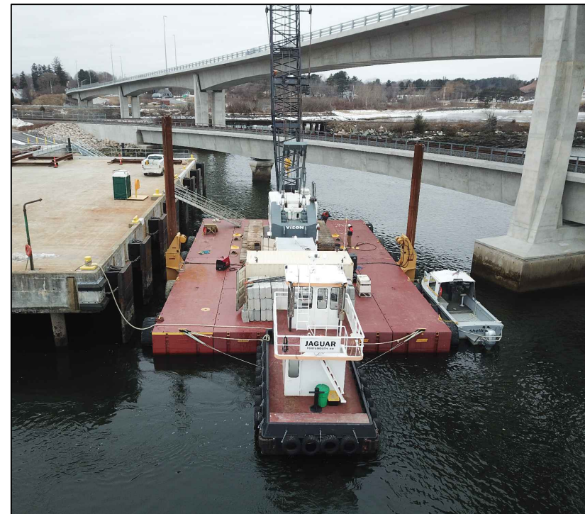
FLOATING DOCK - NEW LOCATION LOOKING SOUTHWEST (A4)
