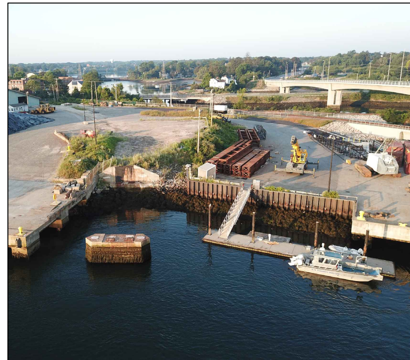
NORTH WHARF EXTENSION LOCATION LOOKING SOUTH
