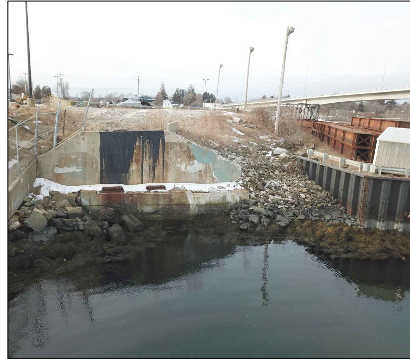
BRIDGE ABUTMENT 13 LOOKING SOUTHWEST (C4)
