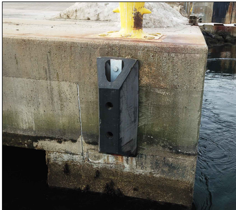
MAIN WHARF - FENDER SYSTEM LOOKING SOUTHWEST
