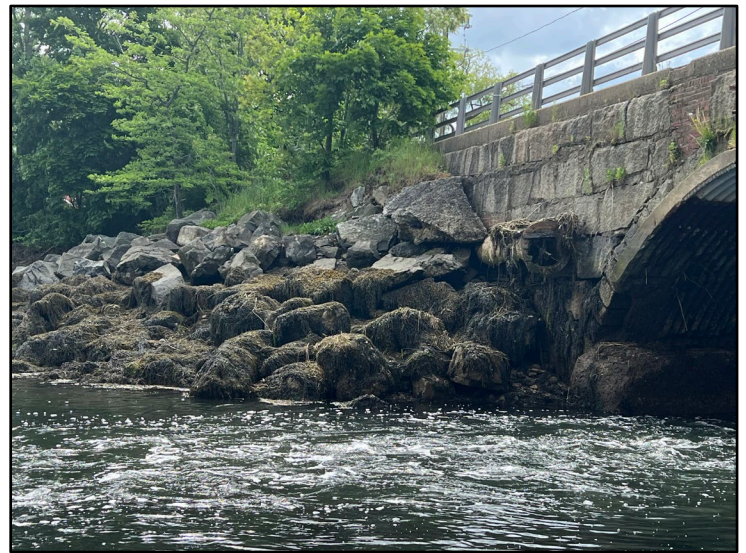
Locations of proposed riprap re-installation with some remaining riprap visible
