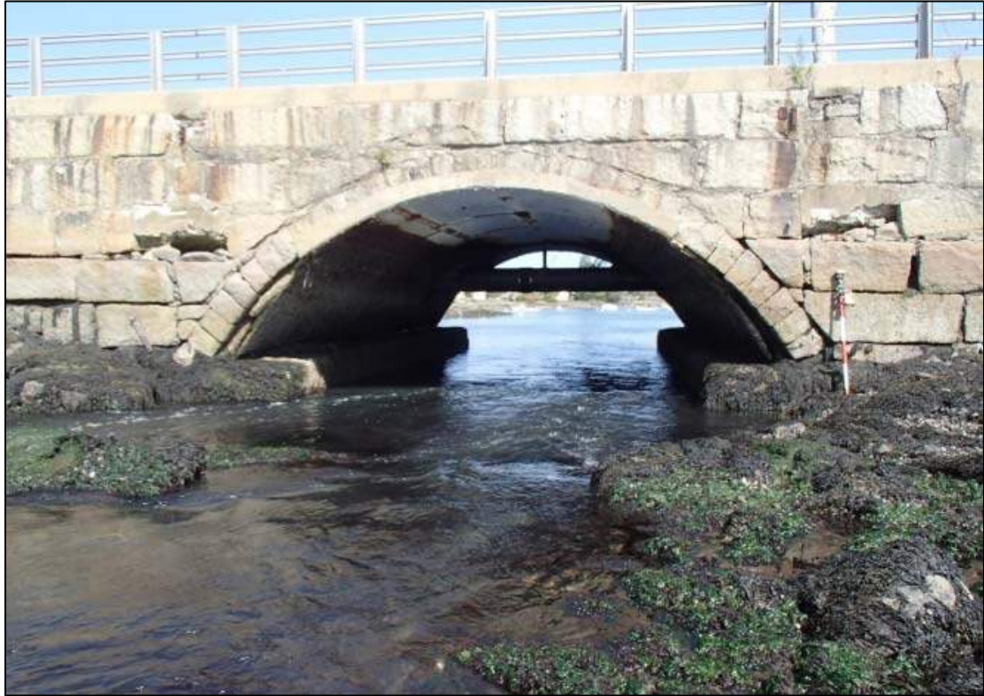
Figure 3 – View north at the existing bridge inlet (09-23-20)
