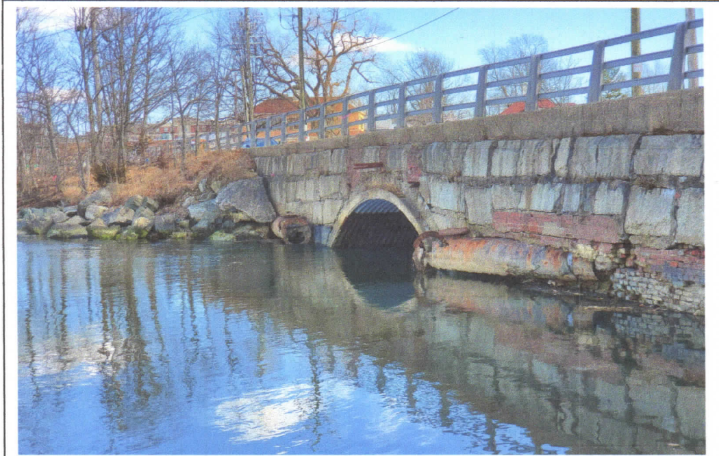
FIGURE 1 Arch Culvert at Maplewood Avenue Over North Mill Pond, Portsmouth, View Southwest of Seaward Side of Culvert from Shoreline (2/28/2020)
