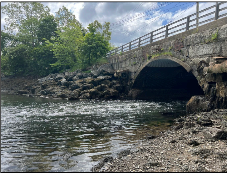
Locations of proposed riprap re-installation with some remaining riprap visible
