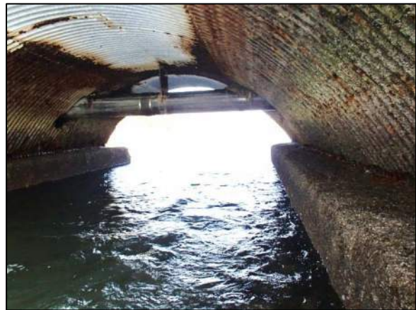
Figure 6 – View north within the existing bridge opening showing the sewer main (09-23-20)
