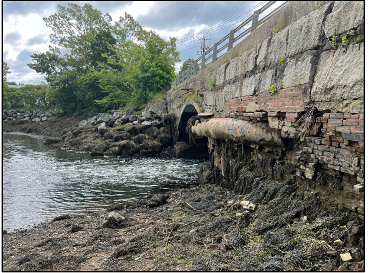
Locations of proposed riprap re-installation
