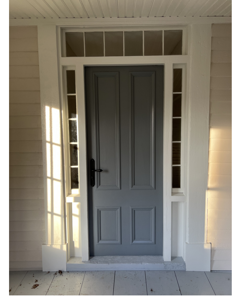
EXISTING FRONT DOOR
