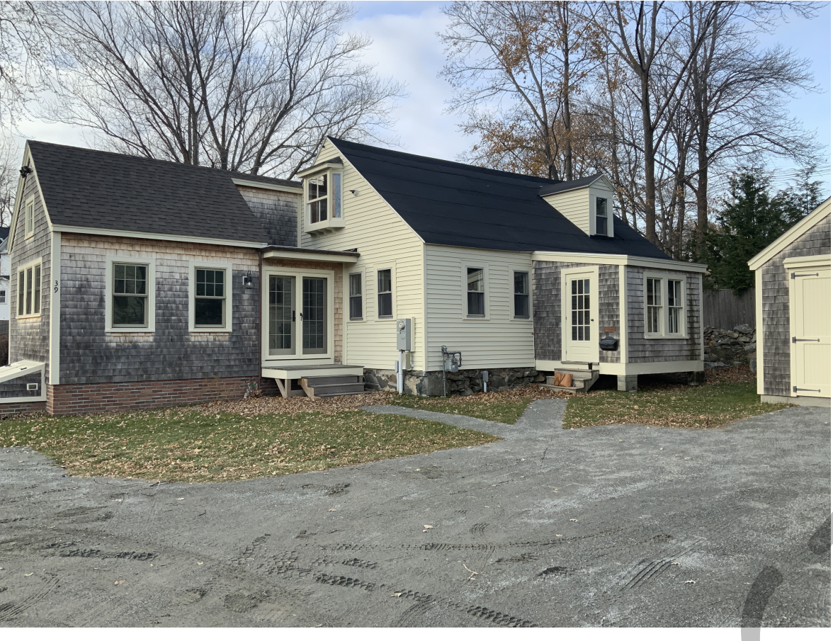
EXISTING FRONT HOUSE
