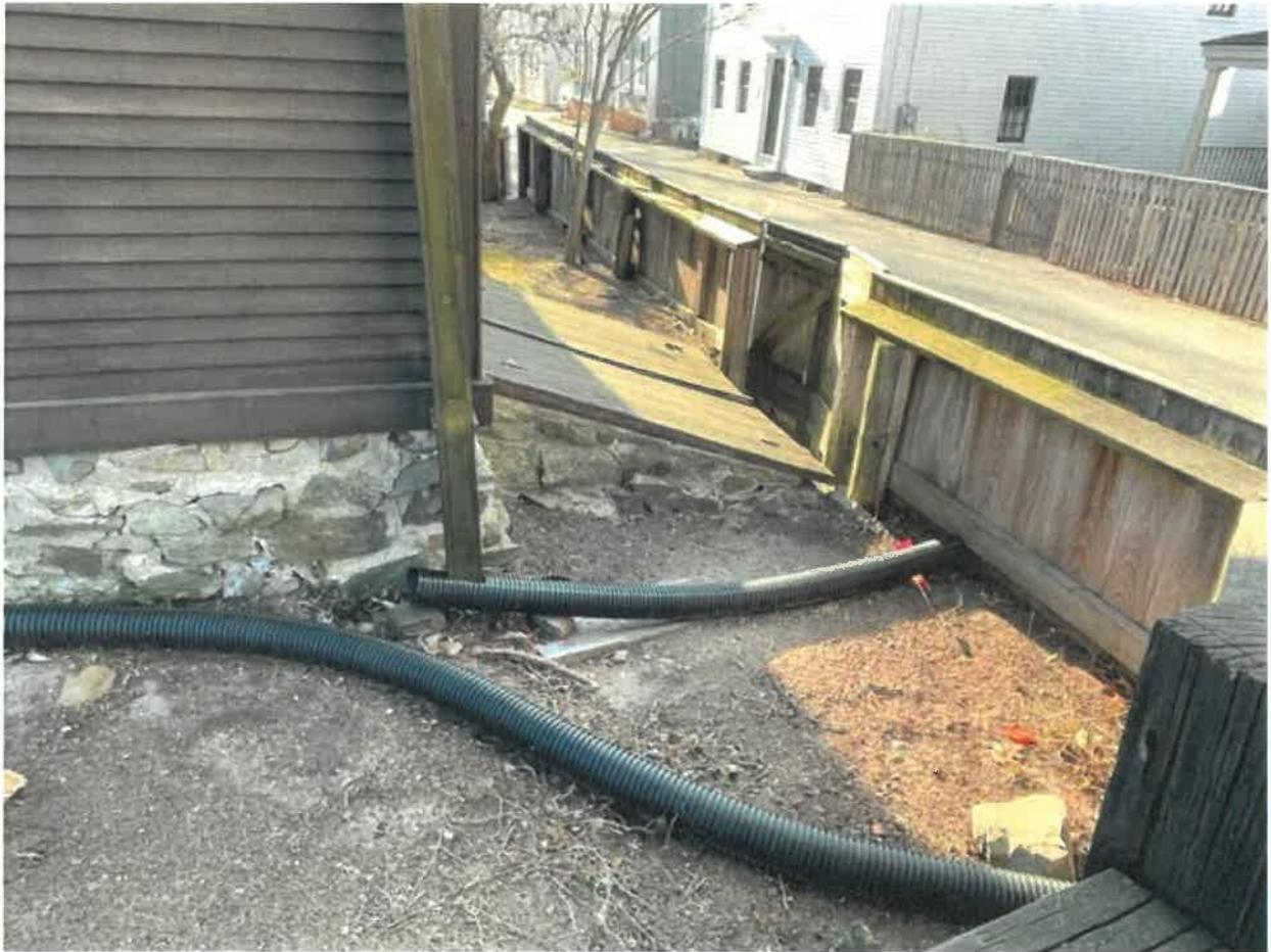
Would like to remove these drainpipes and excavate a new underground drainage pipe with crushed stone and rubber membrane under the surface.
