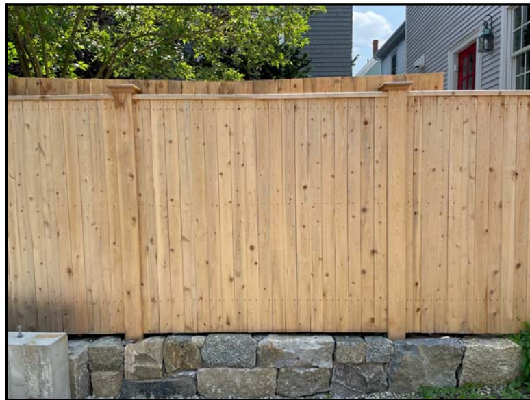
NEW FENCE AT PROPERTY LINE (IMAGE ABOVE), CONDENSER SCREENING TO MATCH
