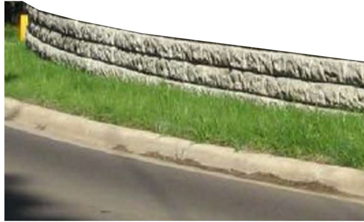
RETAINING WALL (APPROVED 10/5/22)
