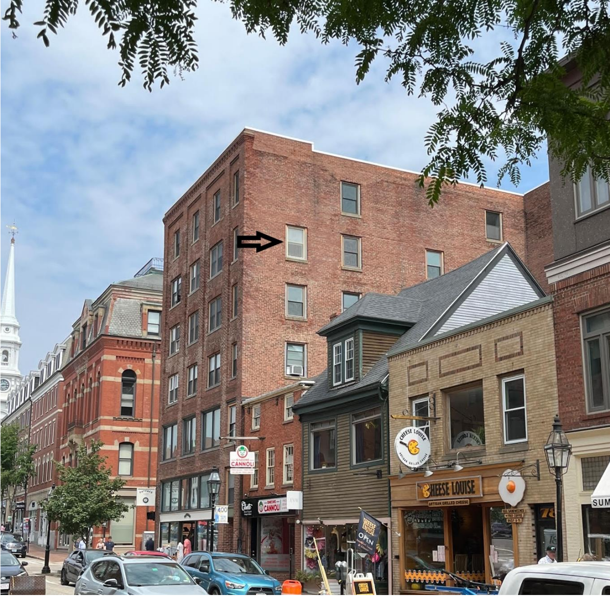
Exterior view of window to be replaced.
