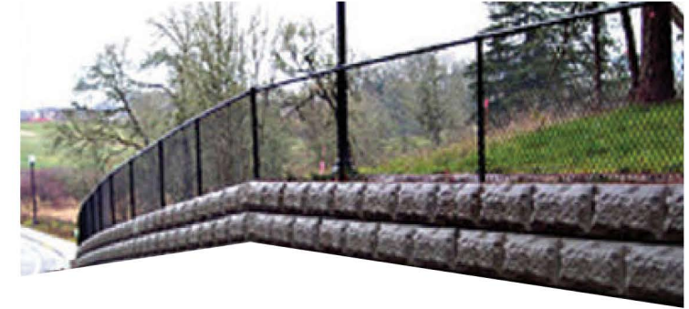
RETAINING WALL (PROPOSED)
