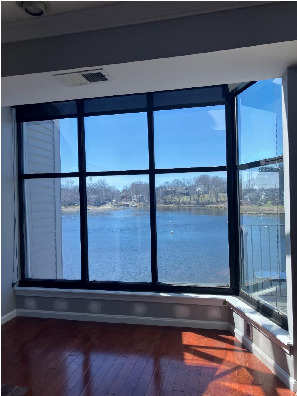
Christopher Goepfert – 500 Market Street Unit 14R – Solarium Window
