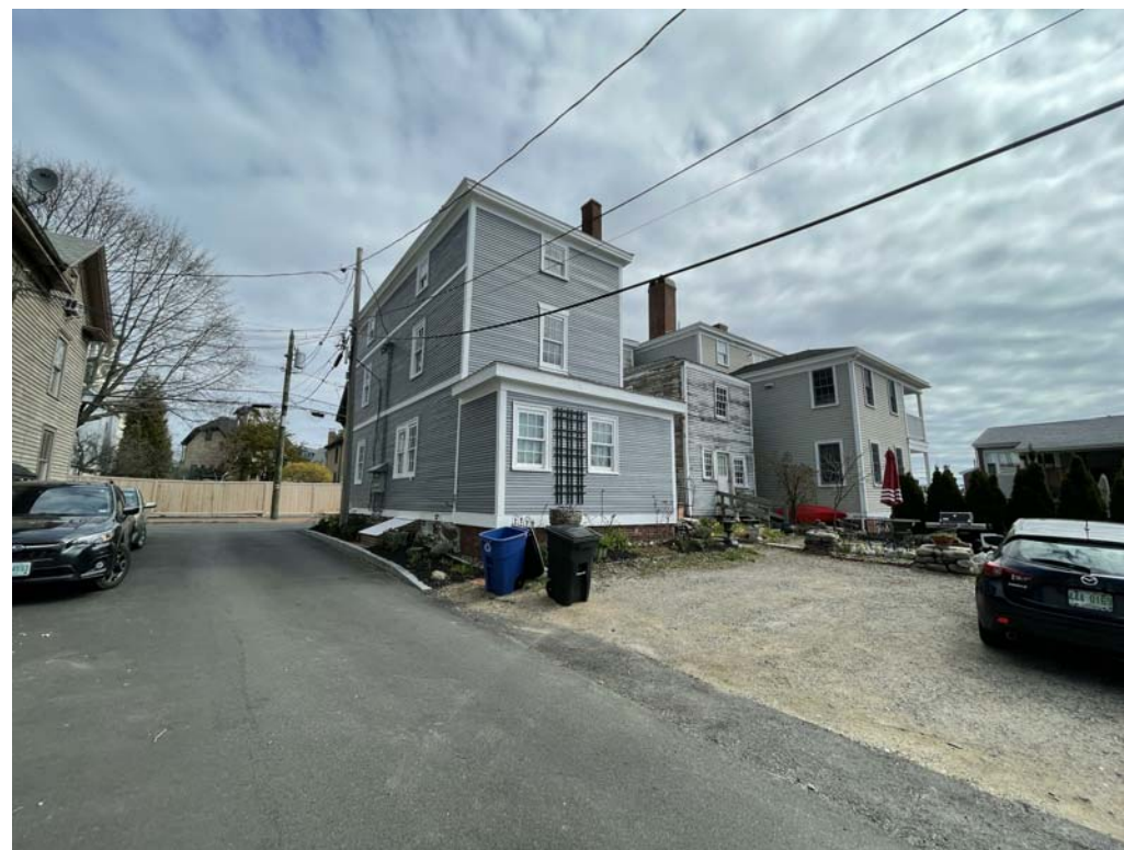
REAR OF BUILDING FROM FRANKLIN STREET
