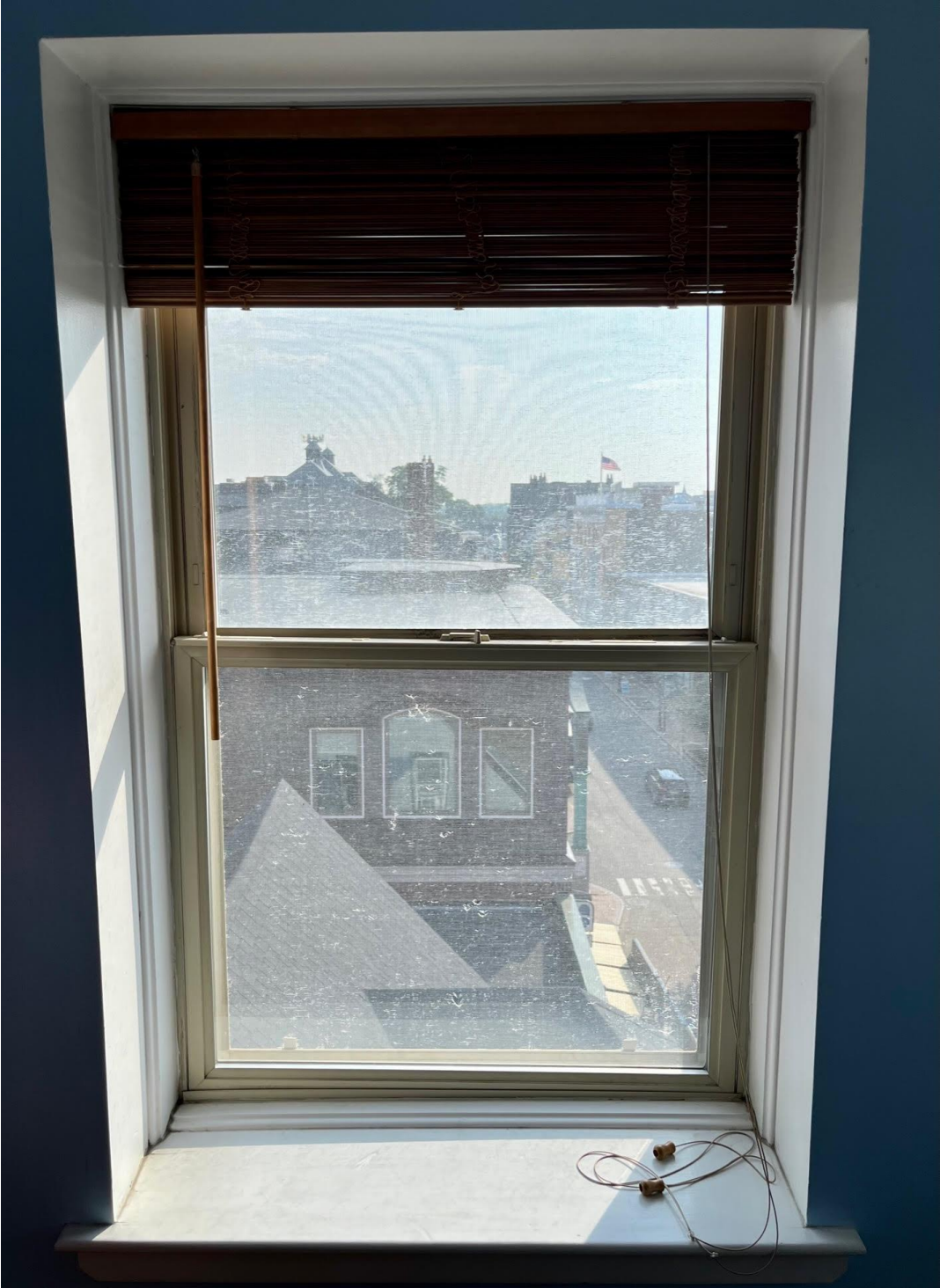
Interior view of window to be replaced.
