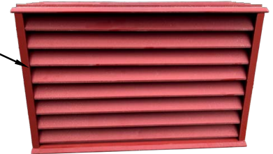
EXAMPLE OF EXIST'G BUILDING VENT PTD.
