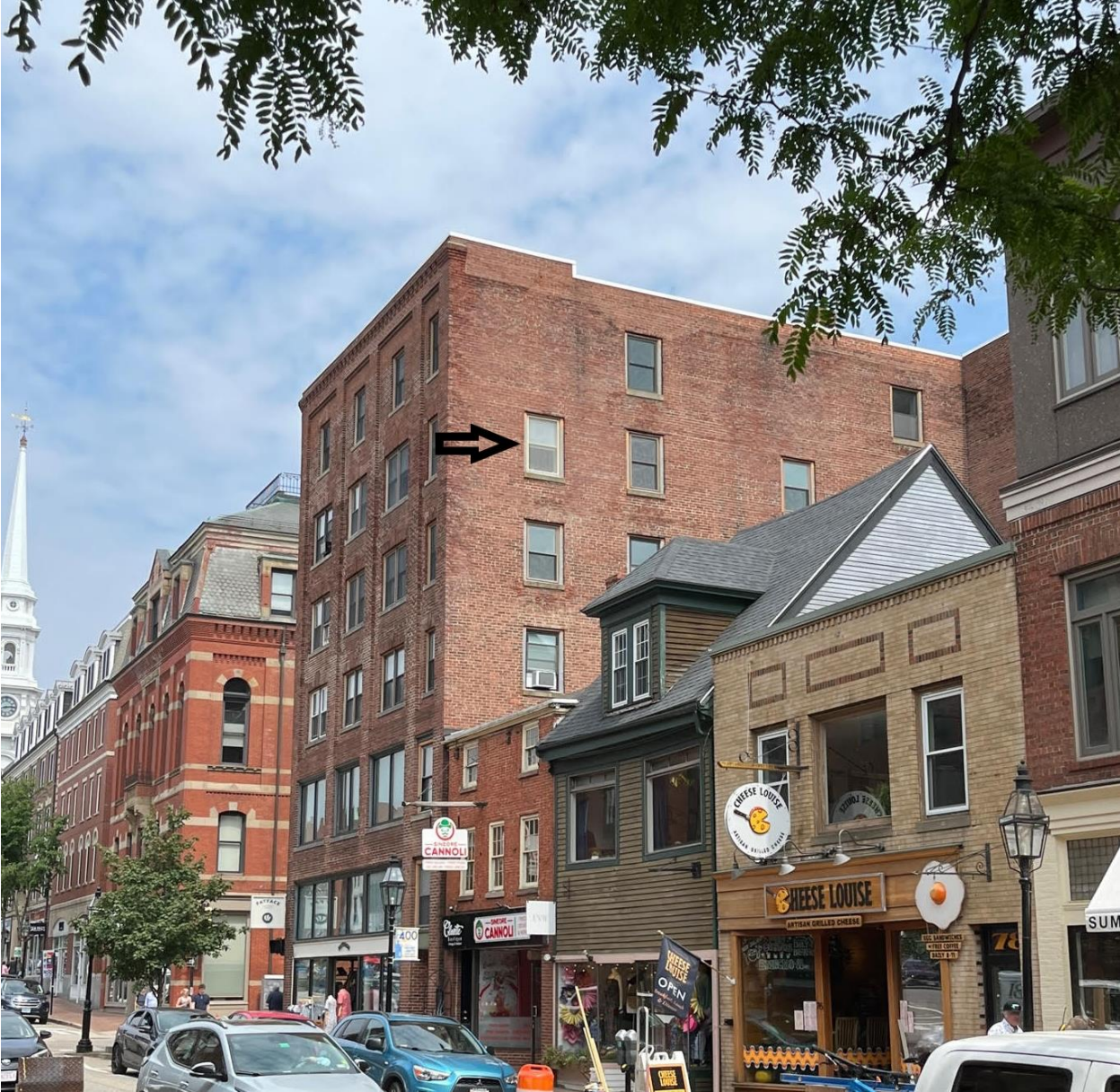
Exterior view of window to be replaced.
