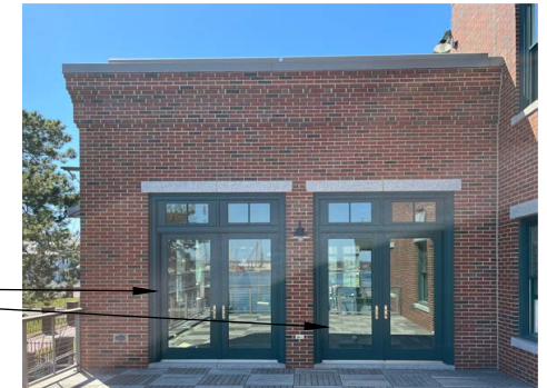
3 UNIT-D 2ND FLR ROOF DECK (EAST/ RIVER ELEVATION)
