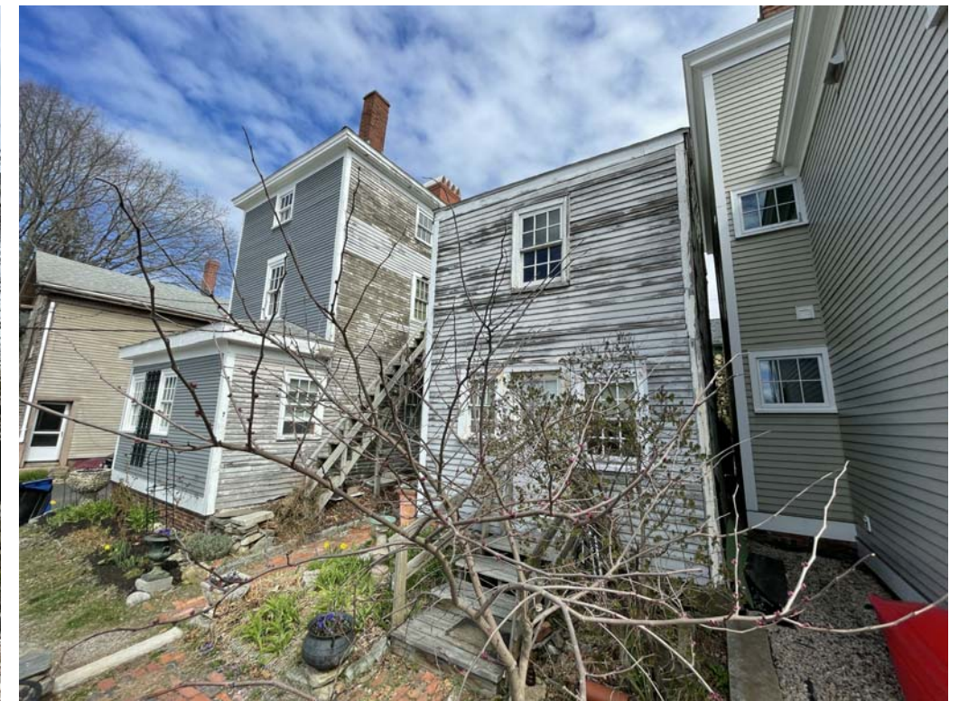
VIEW OF EXISTING SOUTHEAST ADDITION
