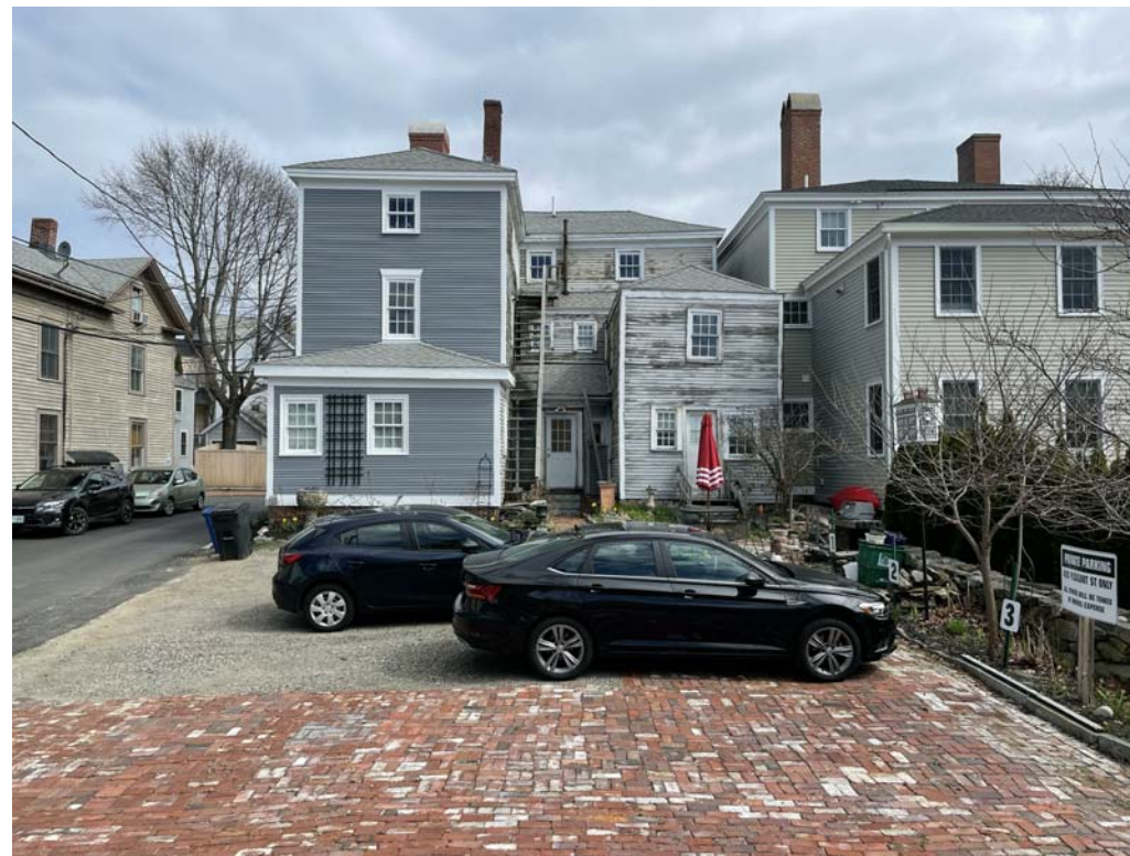
VIEW FROM 420 PLEASANT STREET PARKING LOT
