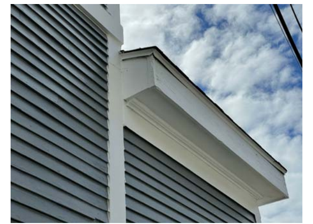
DESIGN INTENT: MATCH EXISTING HIP ROOF EAVE AND SOFFIT WOOD TRIM, WOOD CORNERBOARDS AND OTHER WOOD TRIM AT PROPOSED ADDITIONS
