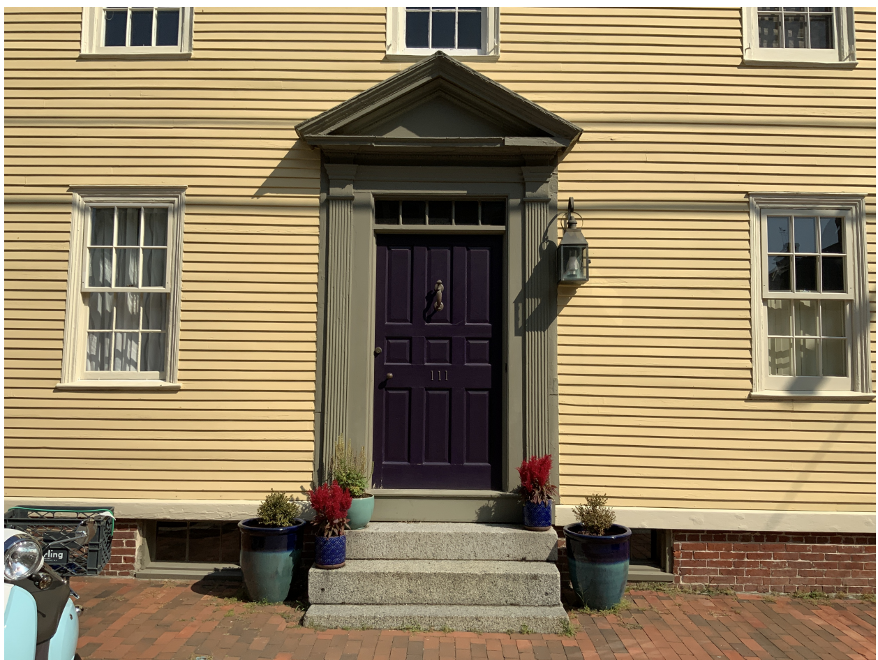
FRONT MAIN DOOR
