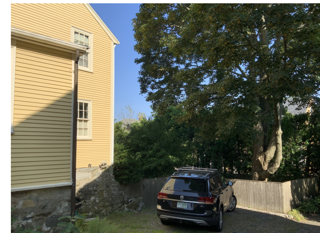
RIGHT SIDE PARKING AREA PROPERTY FENCE
