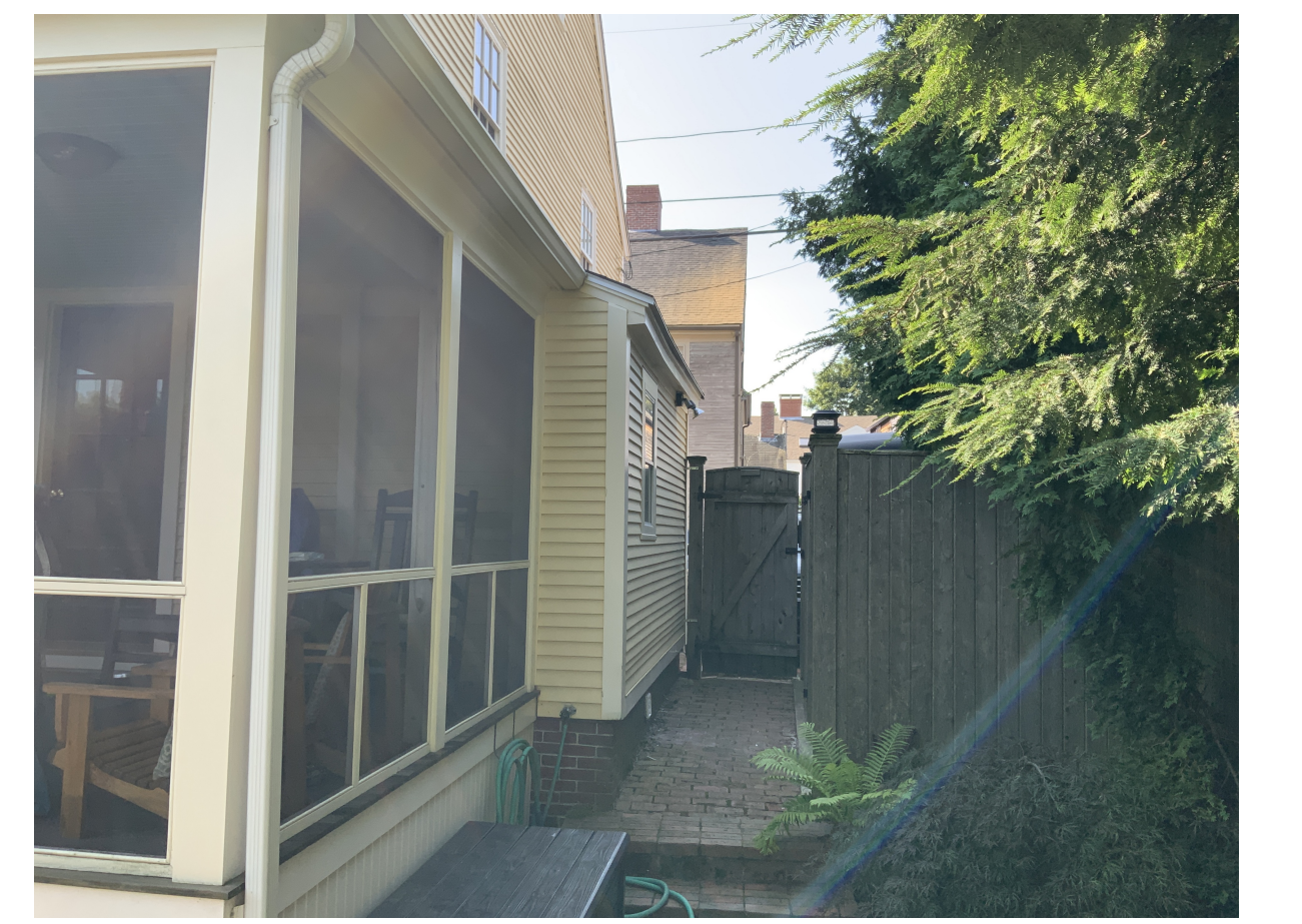
LEFT SIDE REAR SCREEN PORCH & STORAGE AREA
