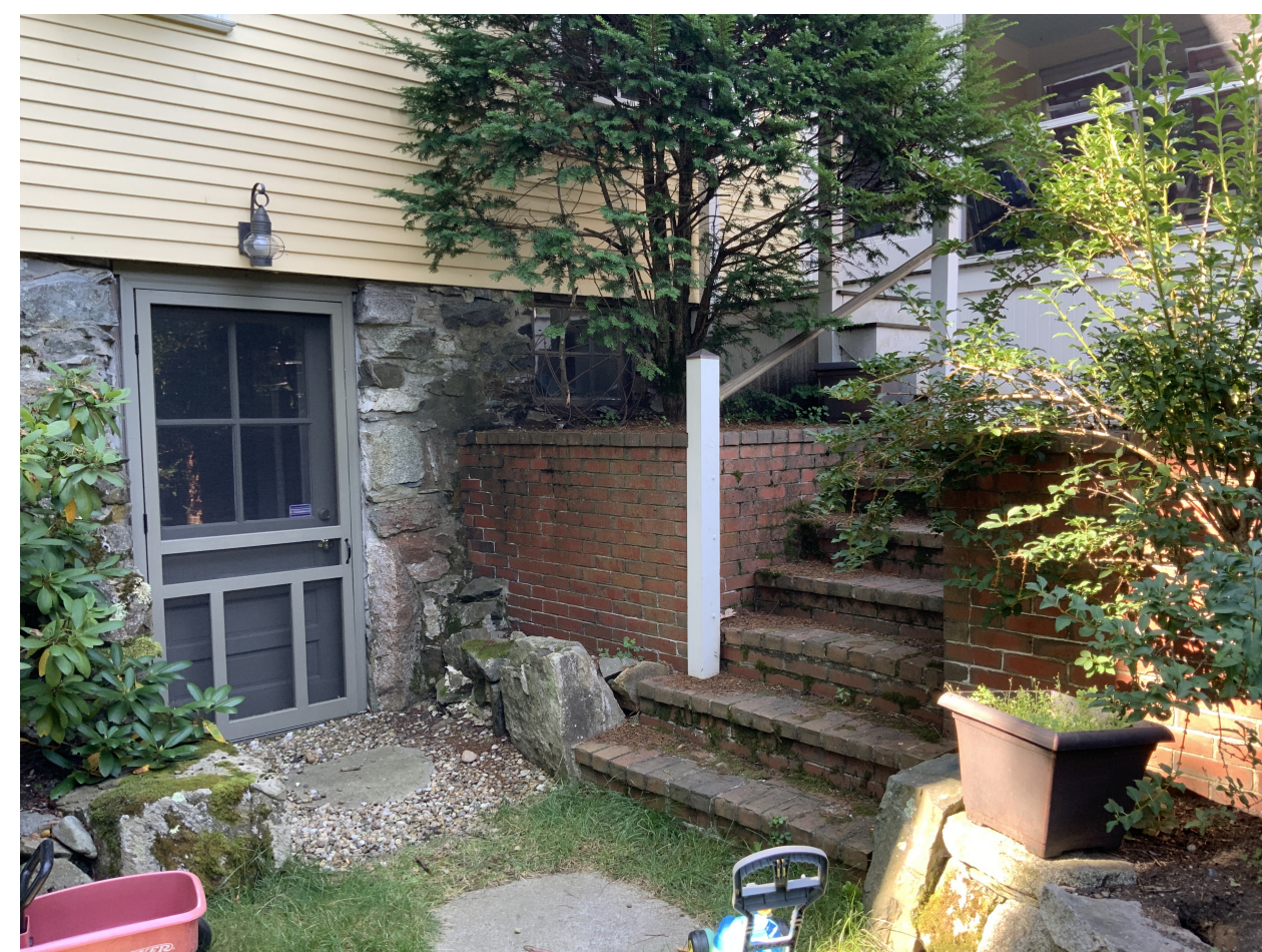
REAR BASEMENT DOOR
