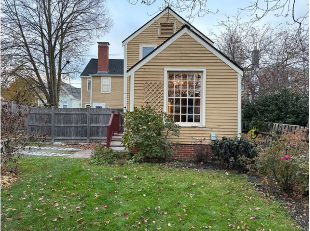
Window to be removed and French door with granite 36"x36" landing and stairs to be intalled.
