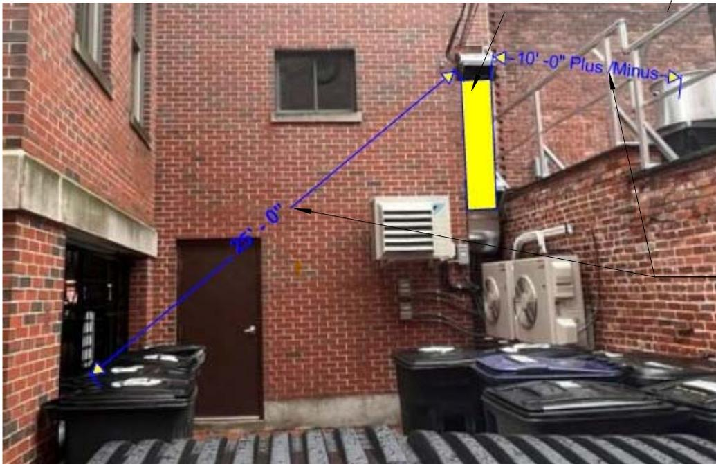
GOOSENECK INTAKE GRILL MUST BE LOCATED 25'-0" MIN. FROM POTENTIAL CAR EXHAUST AND 10'-0" MIN. FROM ADJACENT EXHAUST FANS
