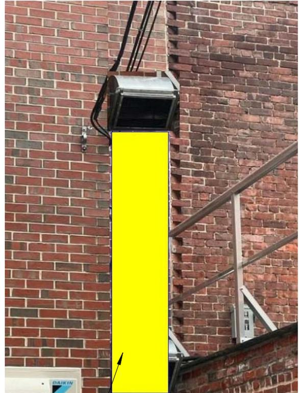
GOOSENECK INTAKE GRILL MUST BE EXTENDED 10'-0" UPWARD TO SATISFY THE MECHANICAL CODE. YELLOW REPRESENTS APPROXIMATE 10'-0" LENGTH OF EXTERIOR DUCT TO BE RUN. DUCTWORK, VENT, AND CONNECTIONS WILL BE PAINTED TO MATCH ADJACENT BRICK.
