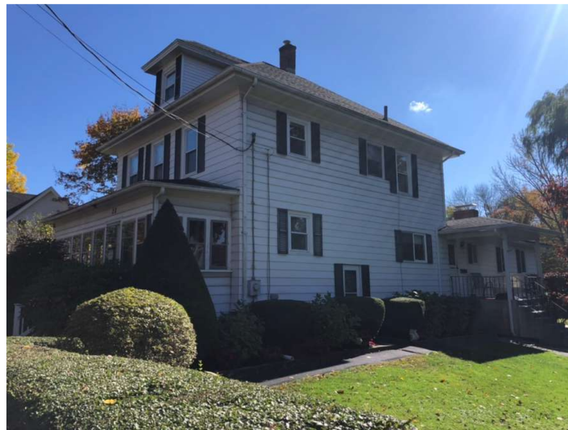
NORTH WEST CORNER
