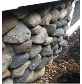
STONES AT EXISTING FOUNDATION
