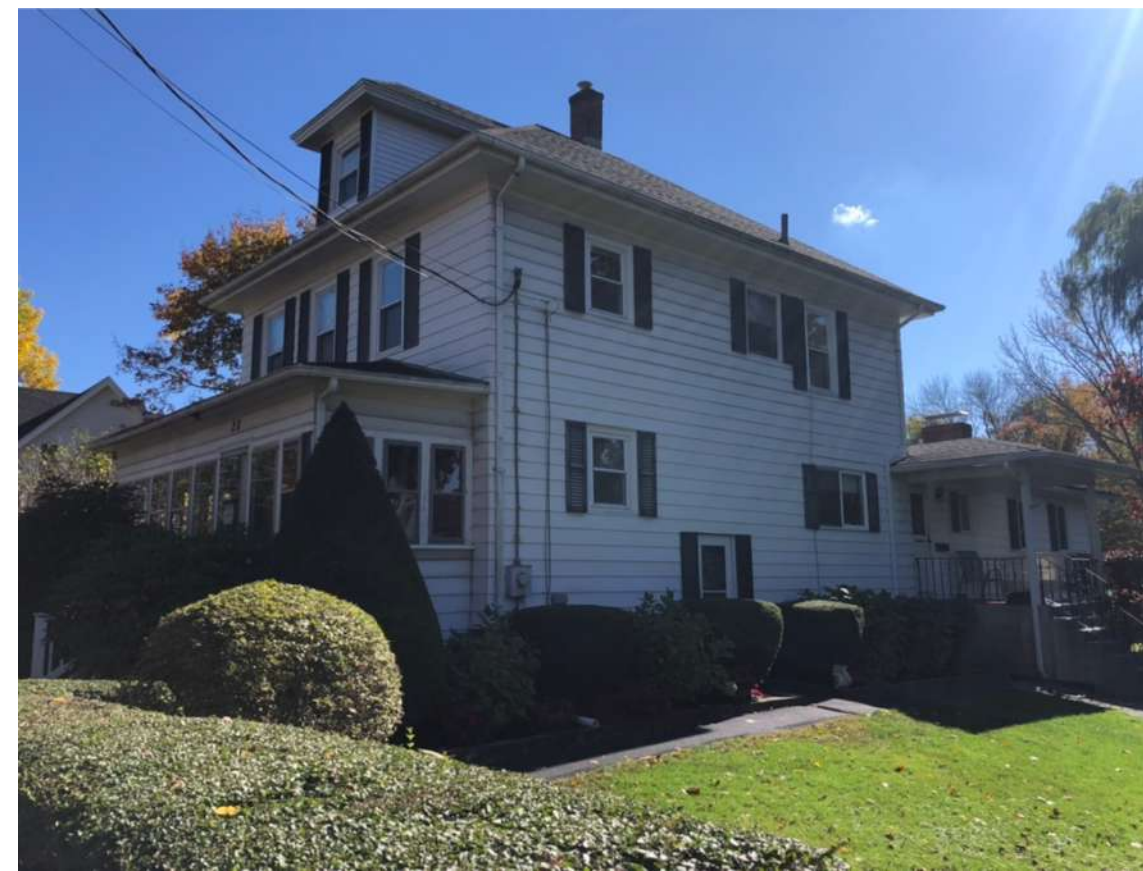
NORTH WEST CORNER
