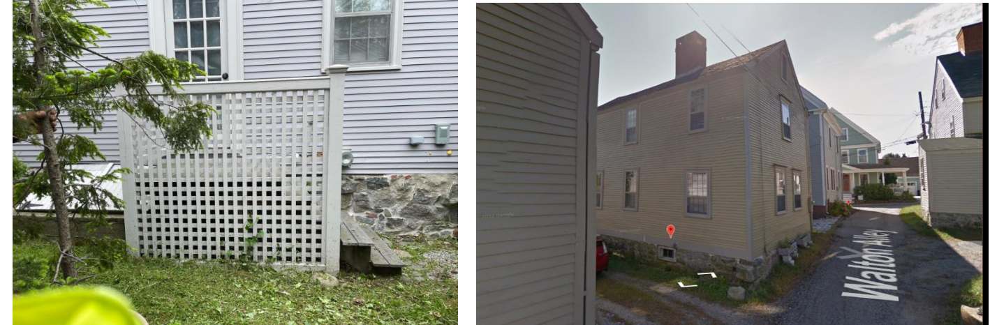
Rear Elevation and Streetscape View
