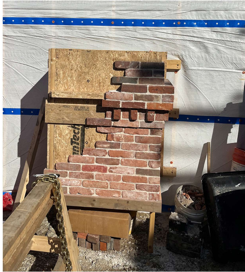
PROPOSED BRICK CHIMNEY MOCKUP
