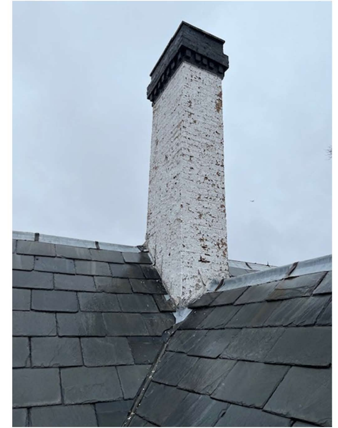
EXISTING BRICK CHIMNEY
