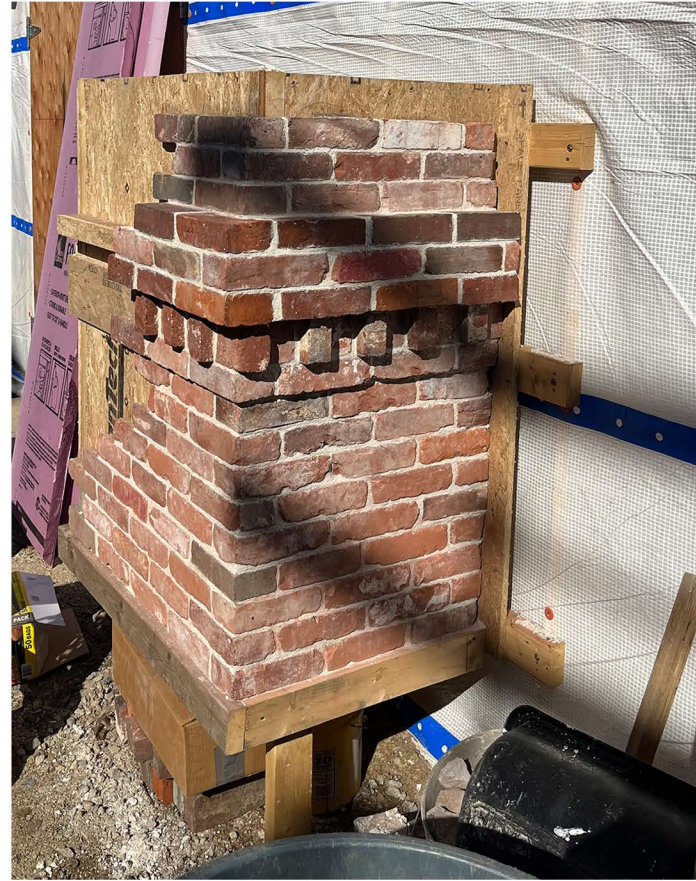
PROPOSED BRICK CHIMNEY MOCKUP
