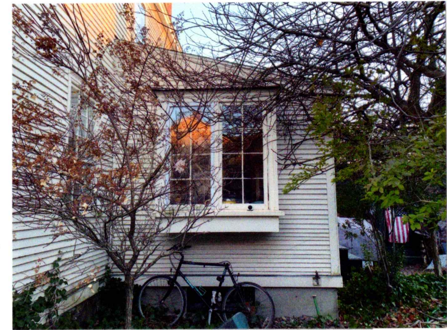
VIEW OF EXIST REAR 1-STORY & BAY
