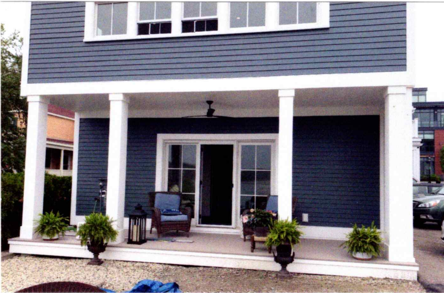
AS BUILT PORCH WITH SQUARE COLUMNS
