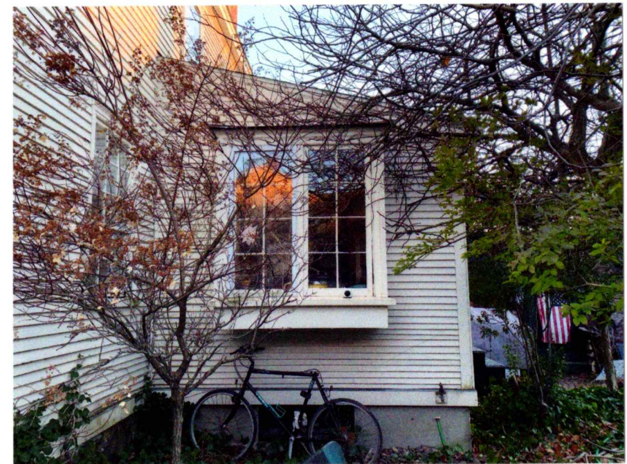
VIEW OF EXIST REAR 1-STORY & BAY
