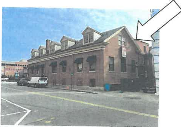
View of building from Hanover Street
