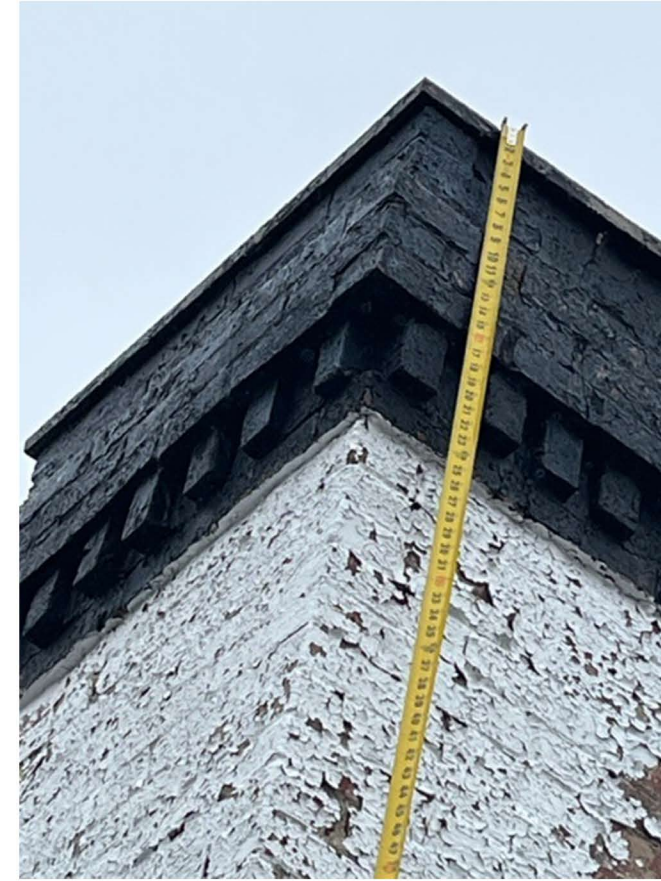
EXISTING BRICK CHIMNEY
