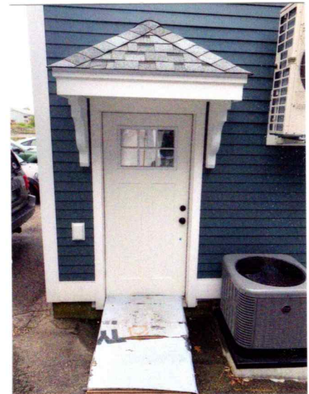
AS BUILT GARAGE SIDE DOOR & ROOF
