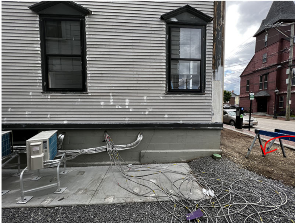
VIEW BETWEEN BUILDINGS AT CONDENSER LOCATION
