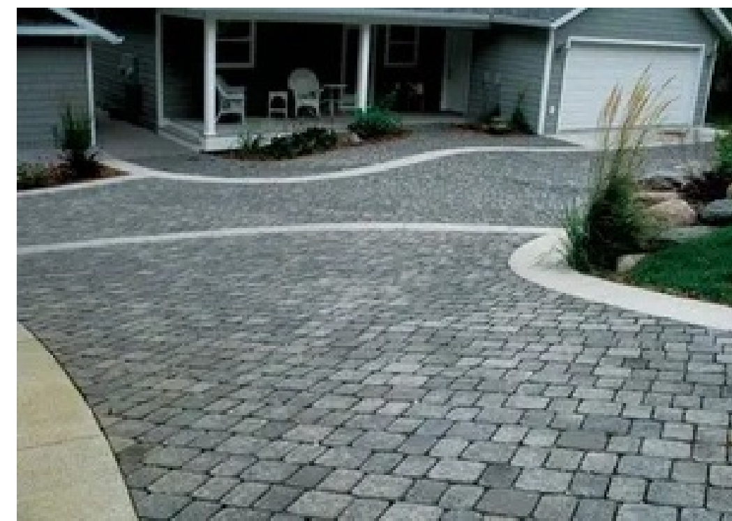
COURTYARD PAVERS GRANITE SQUARE POROUS INSTALLATION
