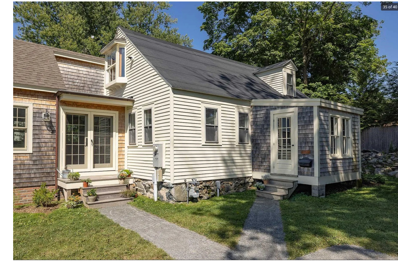
EXISTING VIEW OF ENTRY AND MUDROOM AREA
