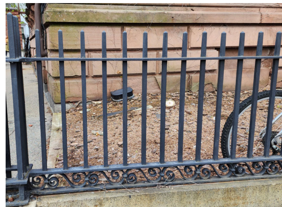
All the exterior railing materials to be metal matching the look and the color of the existing railing
