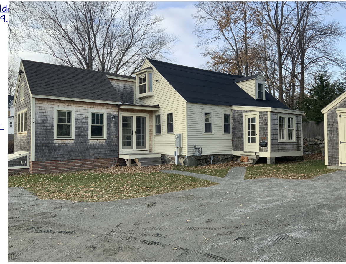
EXISTING FRONT HOUSE
