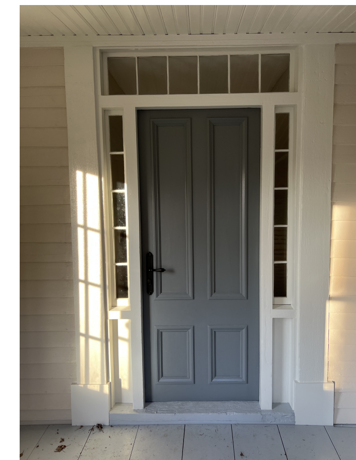
EXISTING FRONT DOOR
