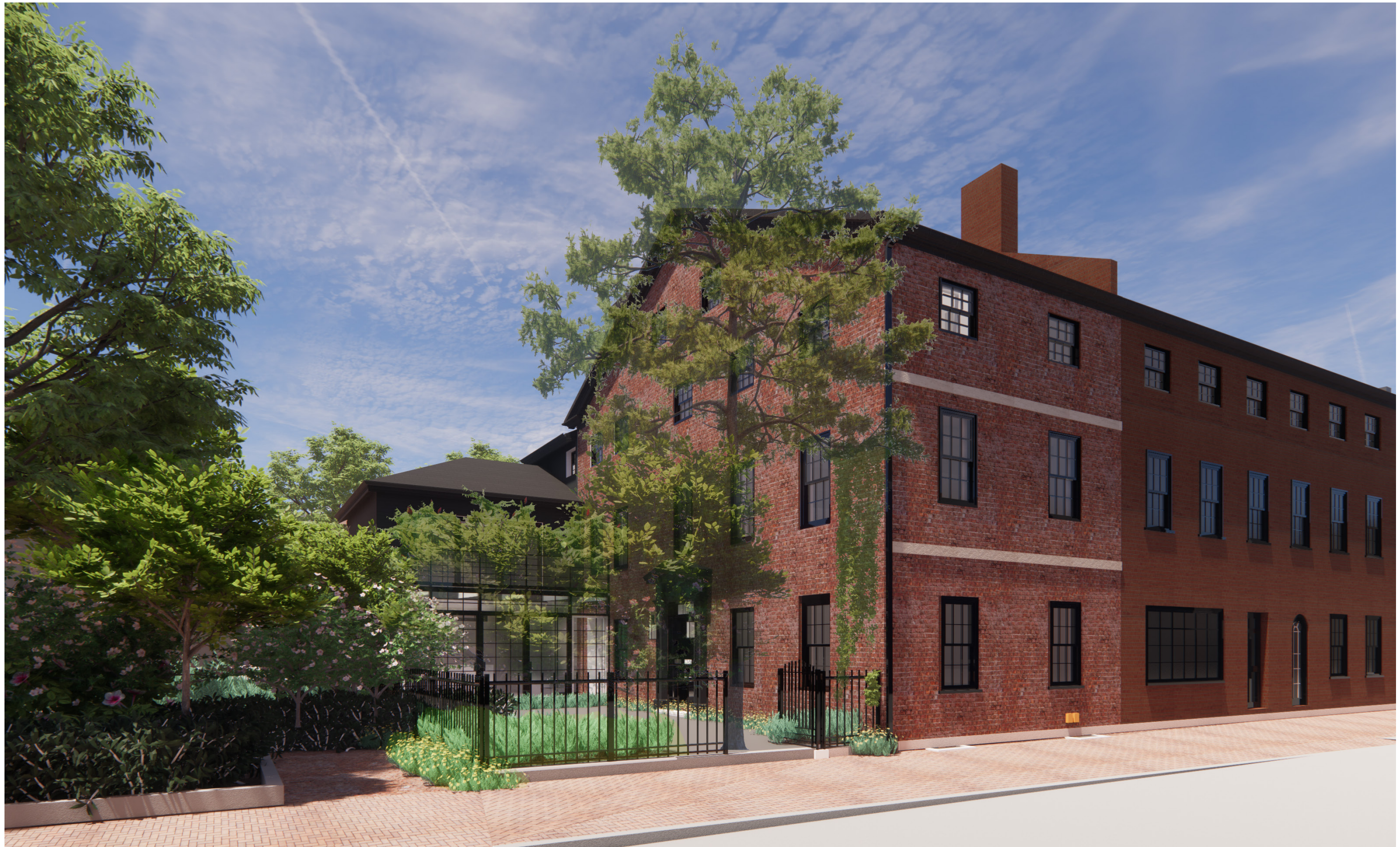
VIEW FROM CORNER OF STATE STREET
