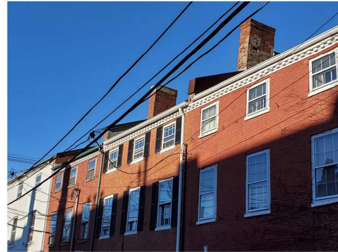
Parapets across Sheafe St
