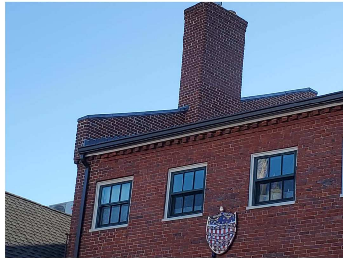
Parapet at opposite end of building
