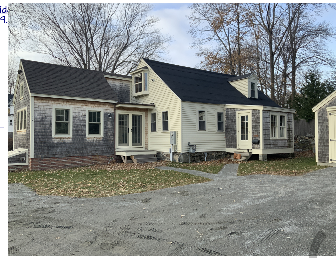
EXISTING FRONT HOUSE
