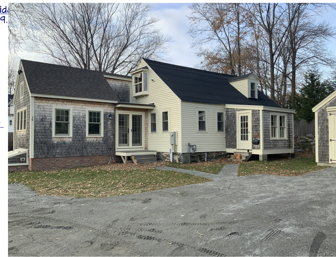
EXISTING FRONT HOUSE
