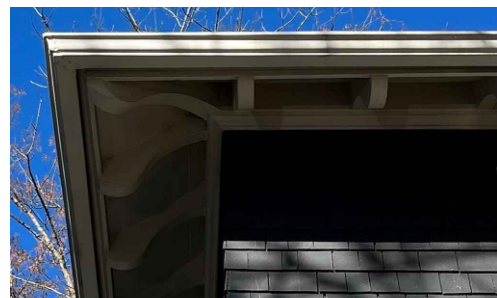
4) ROOF SWEEP AND RAFTER TAILS [FROM BELOW]
