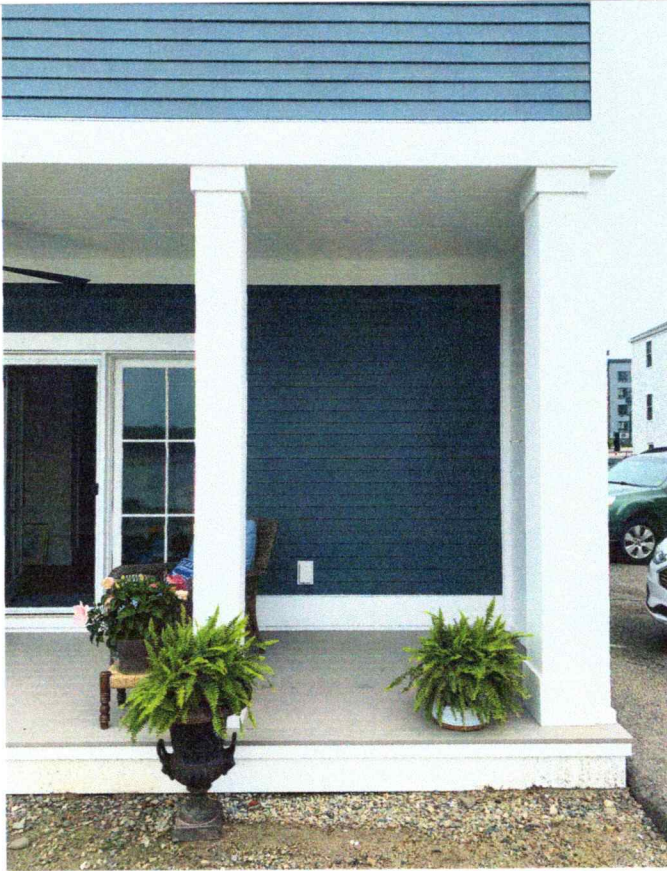
AS-BUILT COLUMN & SCREENING
