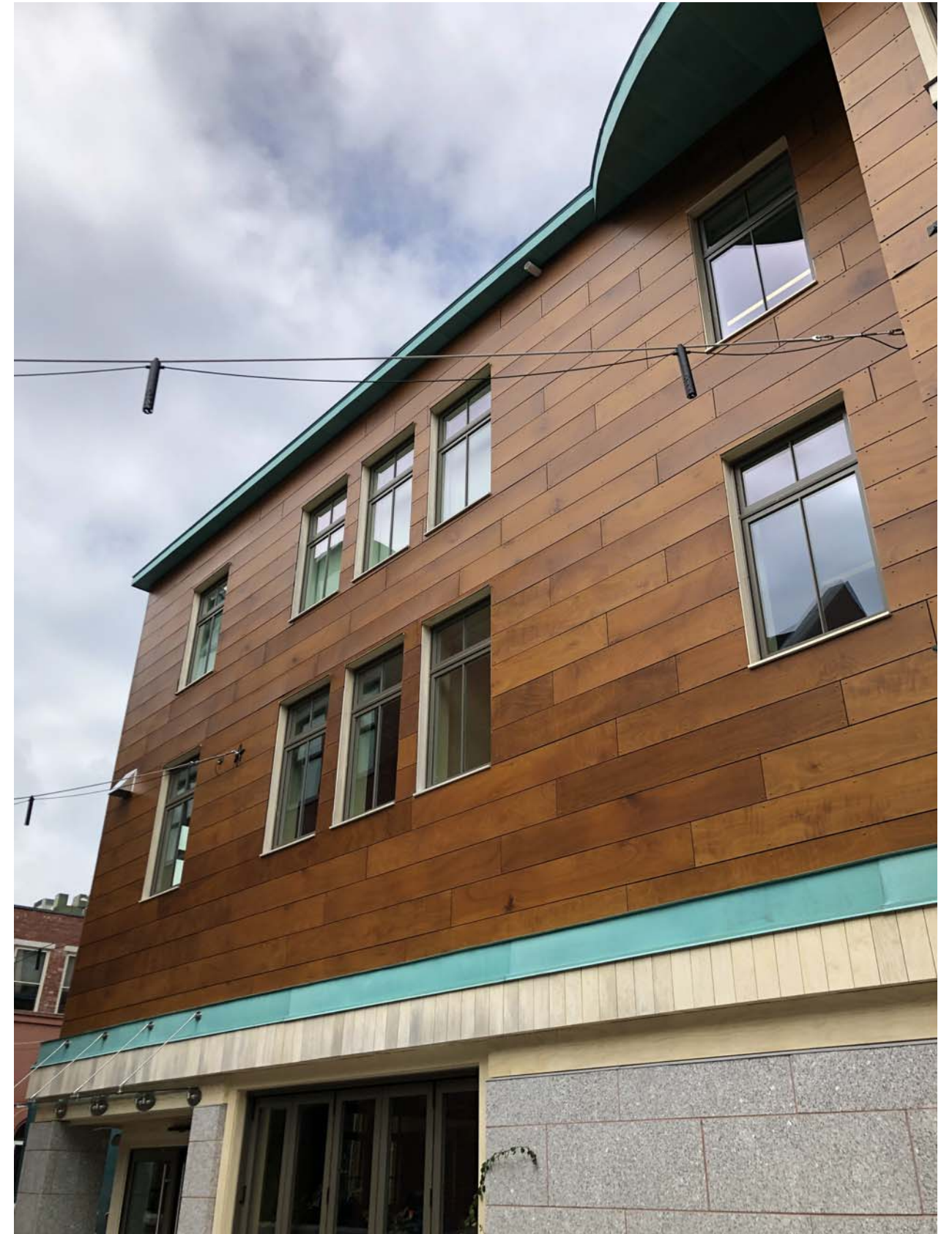
AS-BUILT TRIM ON SOUTH AND WEST FACADES
