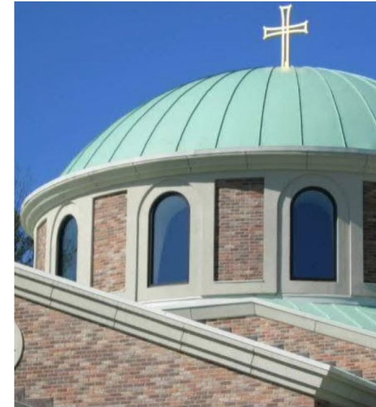
MEMBRANE ROOF WITH SIMULATED STANDING SEAM
