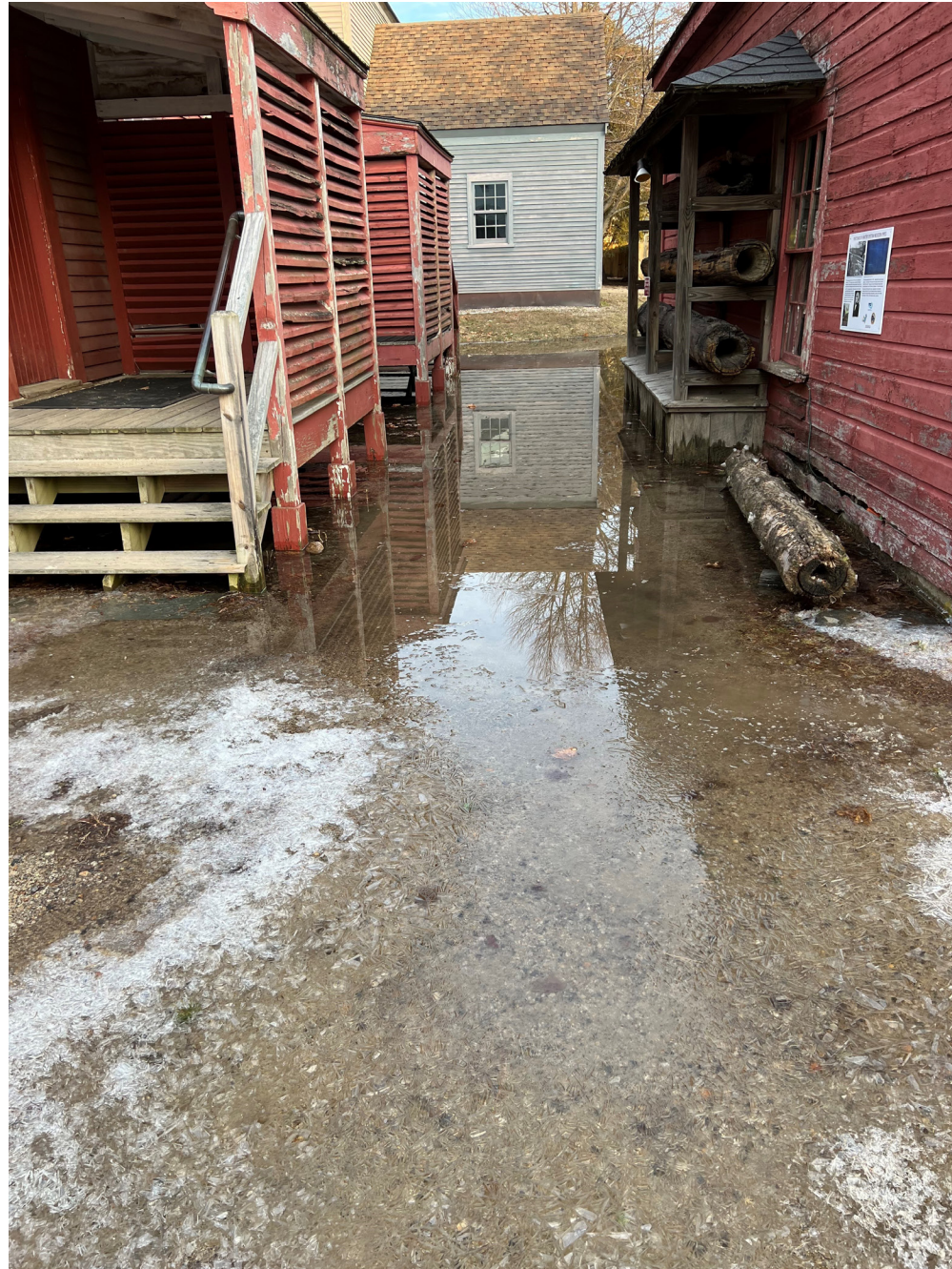
FLOODING AT PENHALLOW REAR
