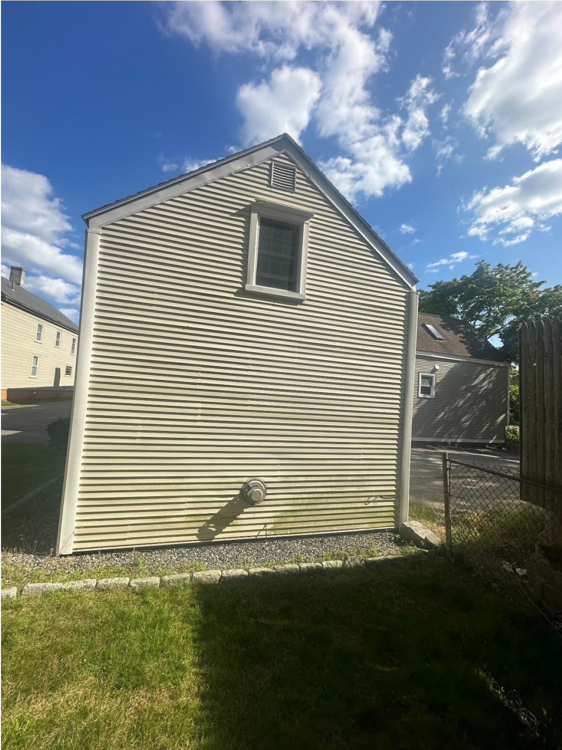
Photo of the existing space where the proposed doorway will be:
