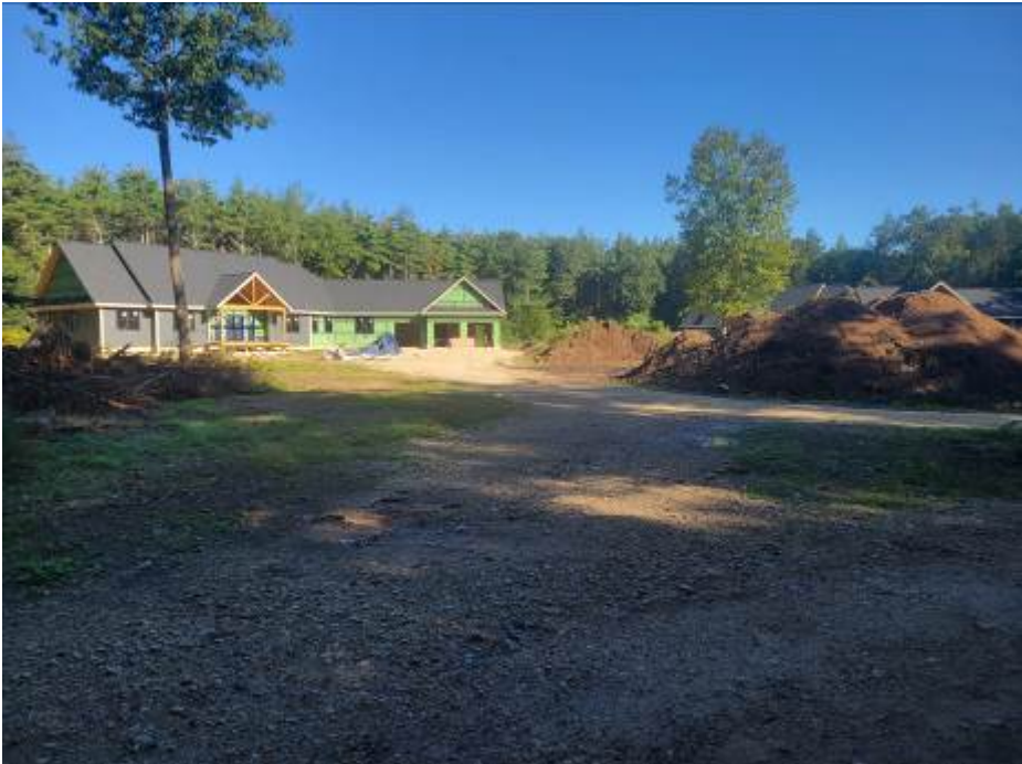
View of 400 Guld Road, Dover, NH – Multiple Residence Development Looking Northwest from Entry Drive - (9/2023)
