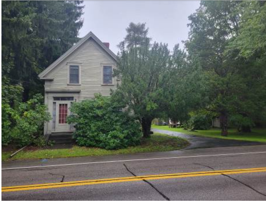
View of Abutting Residence to the South of the Subject Property Looking East - (9/2023)
